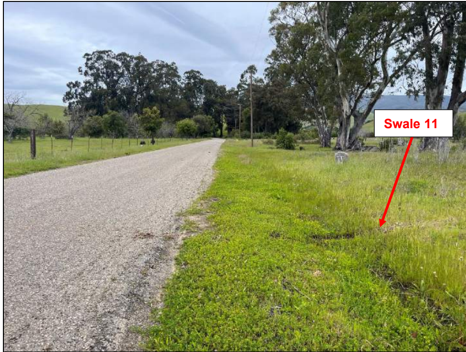
Photo E-5. View looking north along lower reach of San Benito Road with eucalyptus groves in background and Swale 11 visible adjacent to road. Photo taken April 28, 2023.
