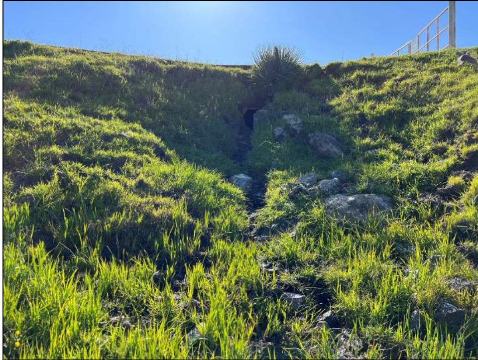
Photo E-17. View of Culvert G from southside of Range Road, looking northeast. Photo taken April 6, 2023.
