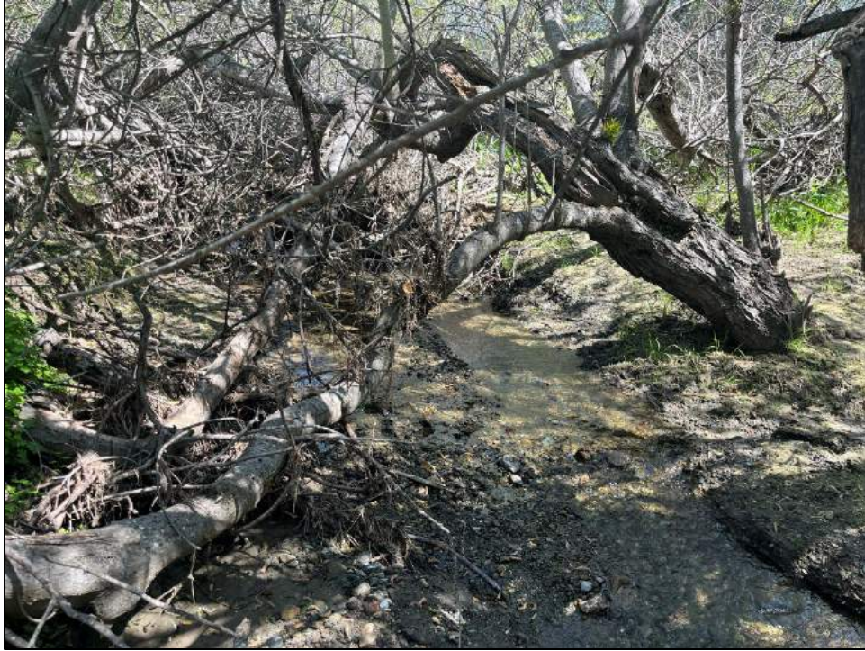
Photo E-13. View south towards Culvert D in flowline of Drainage 9. Oak trees and willows may be removed at this location to facilitate culvert improvements. Photo taken April 6, 2023.
