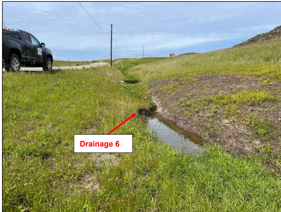
Photo E-11. View west of Drainage 6 running parallel to Range Road. Photo taken April 6, 2023.
