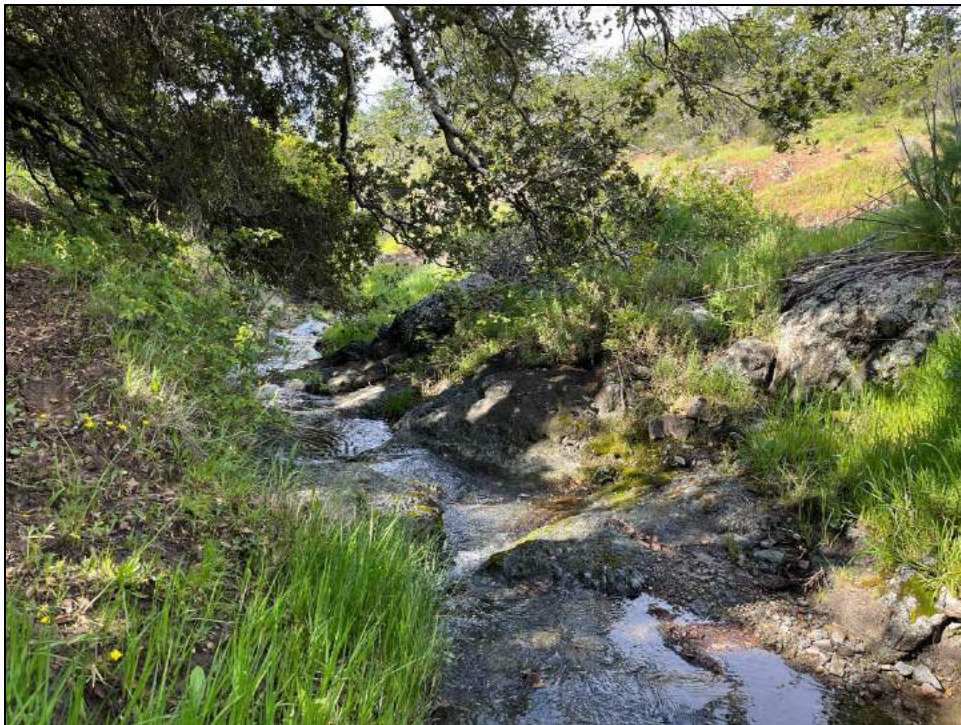
Photo E-14. View north of Drainage 9 downstream of Culvert D. Photo taken April 6, 2023.
