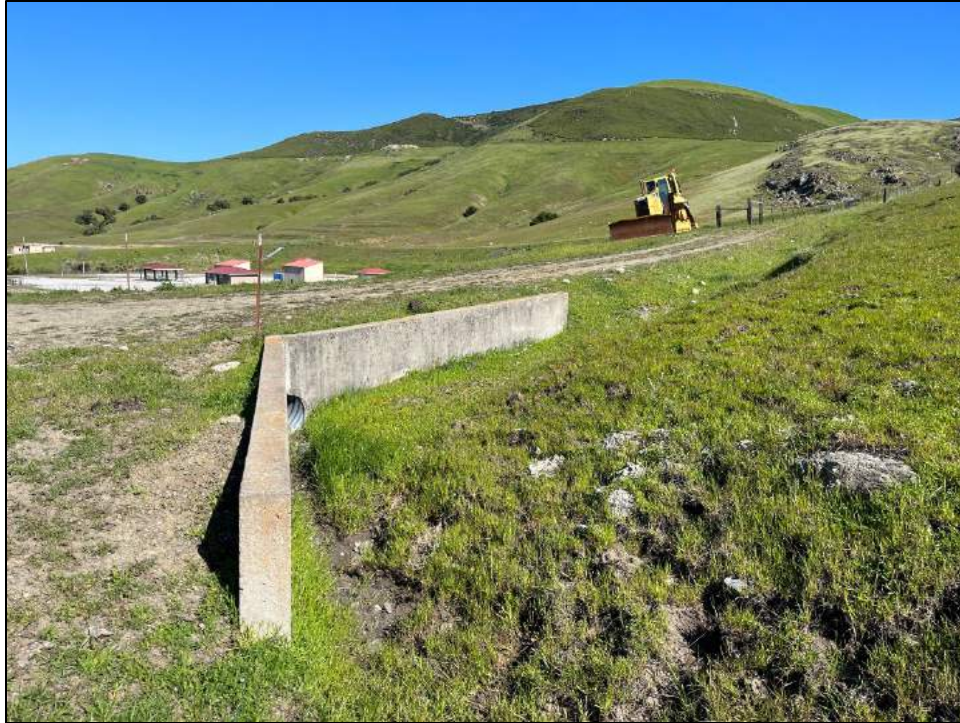
Photo E-15. View west of Culvert F headwall. Non-jurisdictional feature. Photo taken April 6, 2023.
