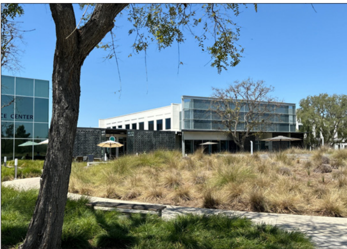
View of on-site office buildings from Susan Street.
