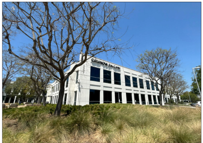
View of on-site northernmost office building from Susan Street.
