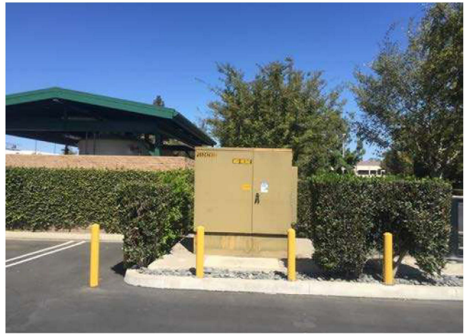
4. View of a typical pad-mounted transformer.
