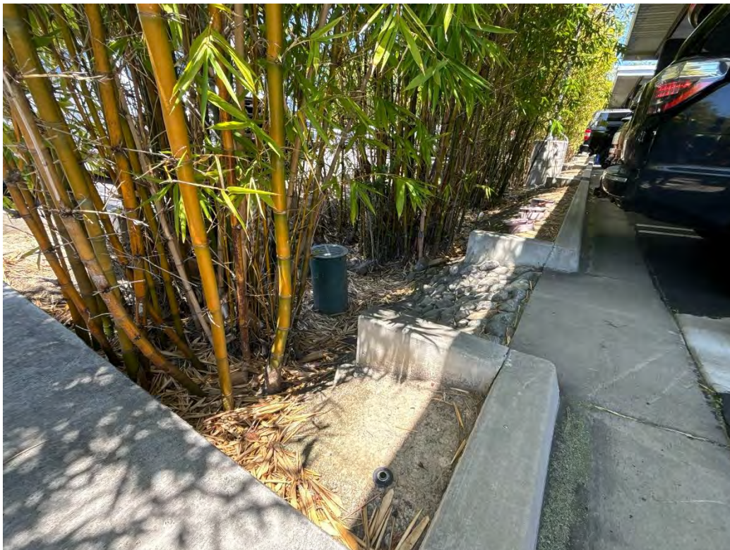
Photograph 8: The west side of the parking lots are generally in rows separated by stalks of bamboo. These areas have been contoured to receive parking lot runoff and represent non-jurisdictional swales.
