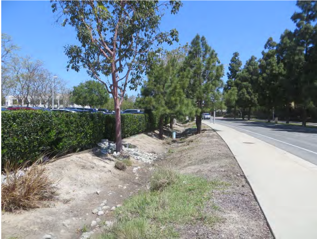
Photograph 11: North-facing view along Susan Street. The eastern side of the parking lot also sends runoff into this non-jurisdictional swale.
