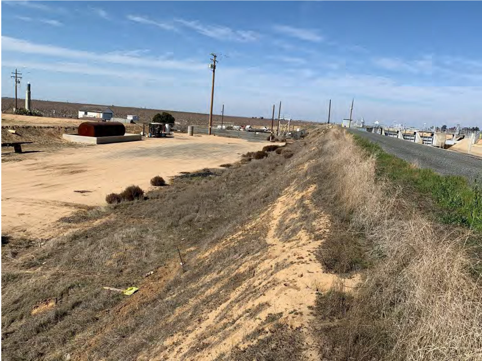
Photo 2: Steep Earthen Embankment Along Access Road
