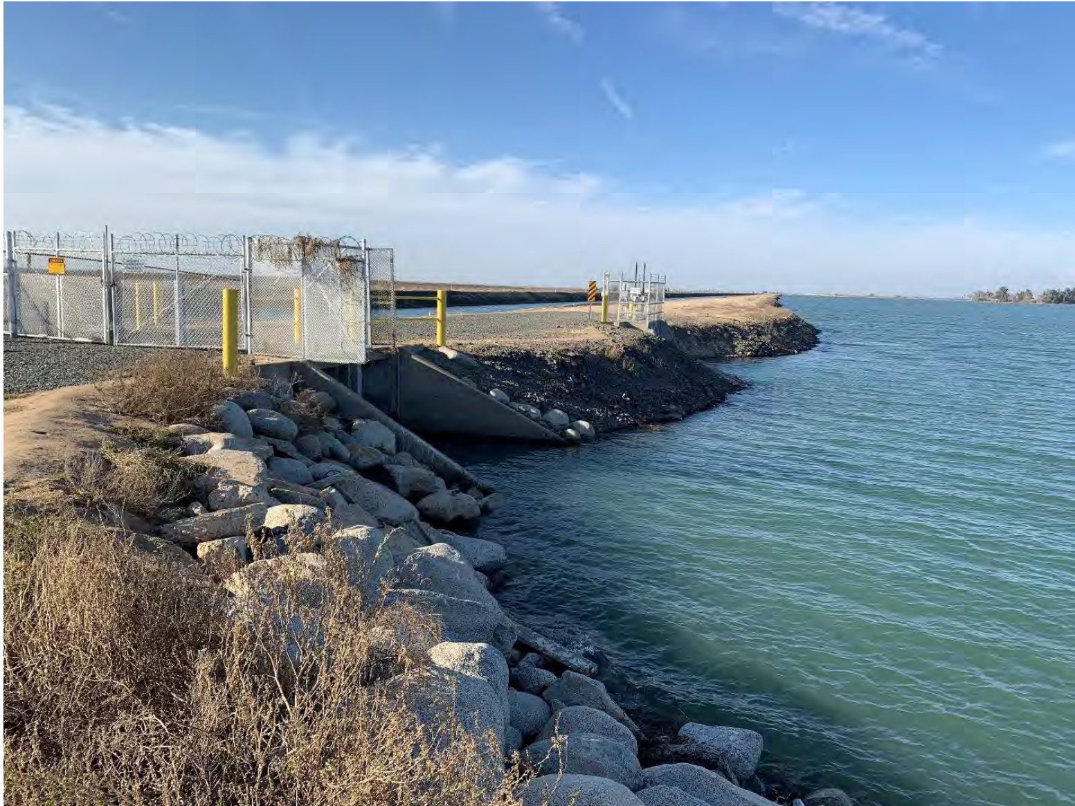
Photo 4: FKC Connection to Lake Woollomes
