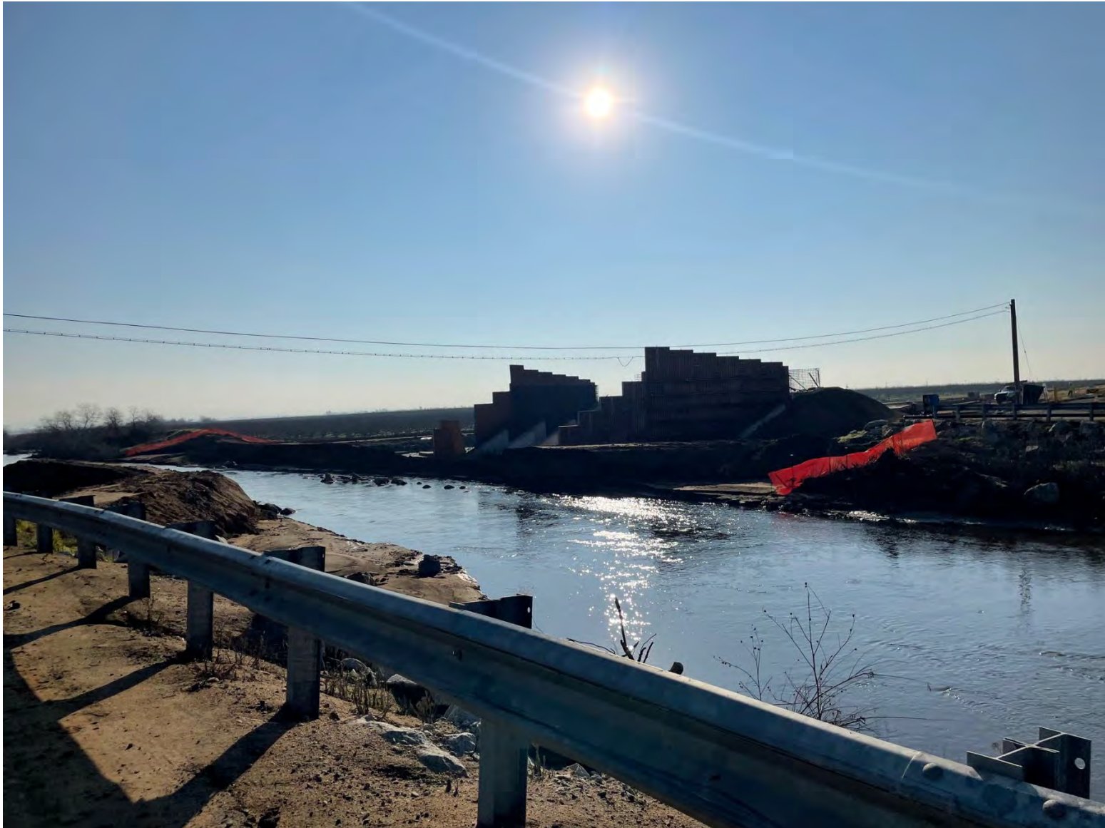
Photo 4: Newly Constructed Siphon Structure on South Side of Deer Creek, East of Friant-Kern Canal Facing southeast
