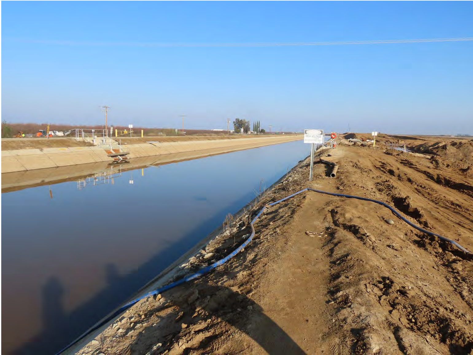
Photo 3: Graded Area East of the Friant-Kern Canal Facing north. Work area is being dewatered (via blue hose) into the Friant-Kern Canal.
