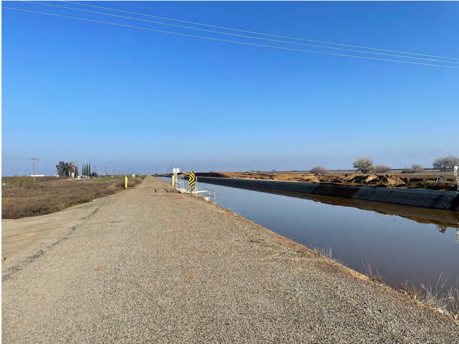
Photo 7: Friant-Kern Canal Infrastructure
