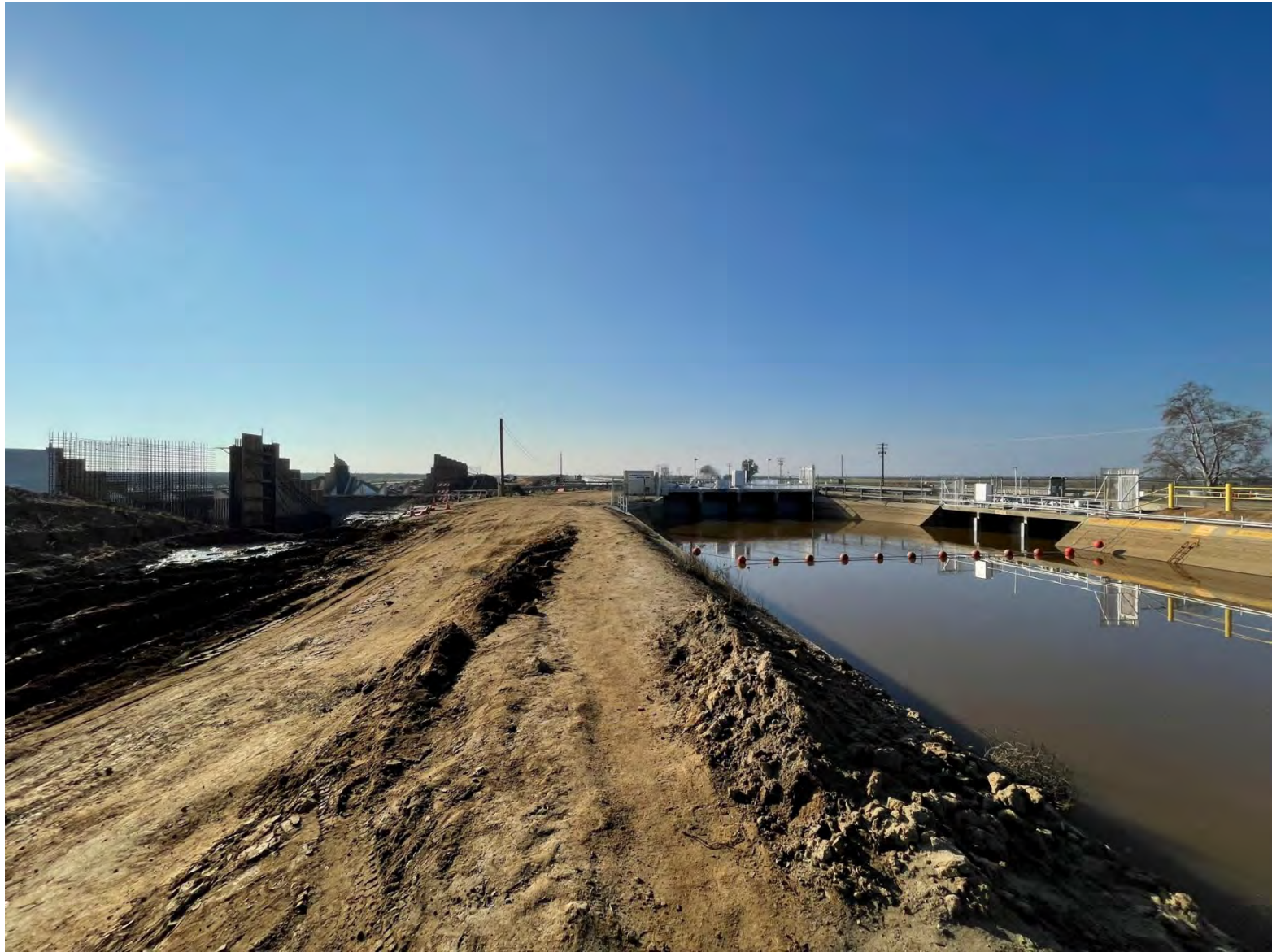
Photo 1: Graded Area East of the Friant-Kern Canal Facing south
