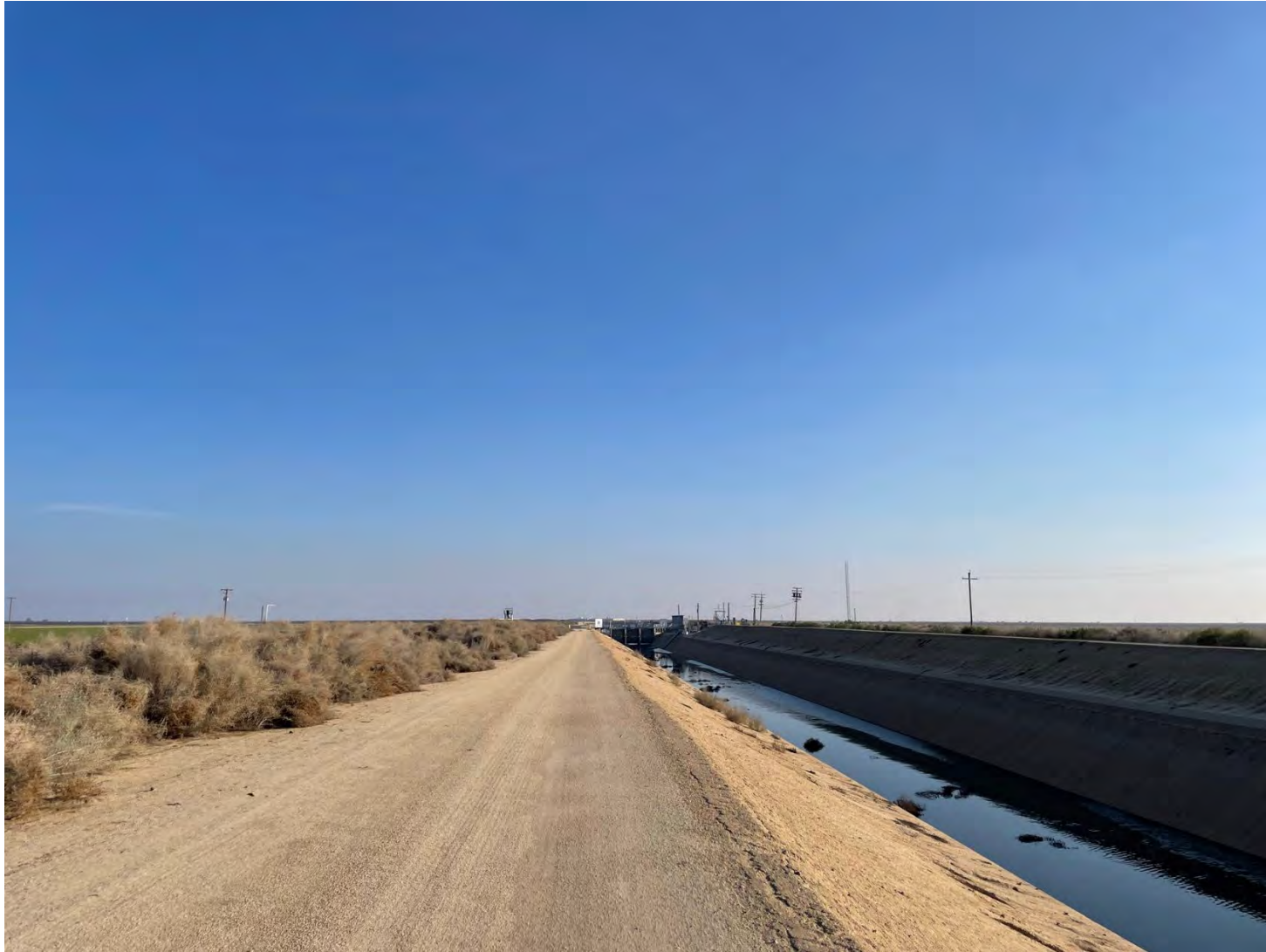
Photo 3: Canal Infrastructure and Gravel-Improved Access Road Facing southeast
