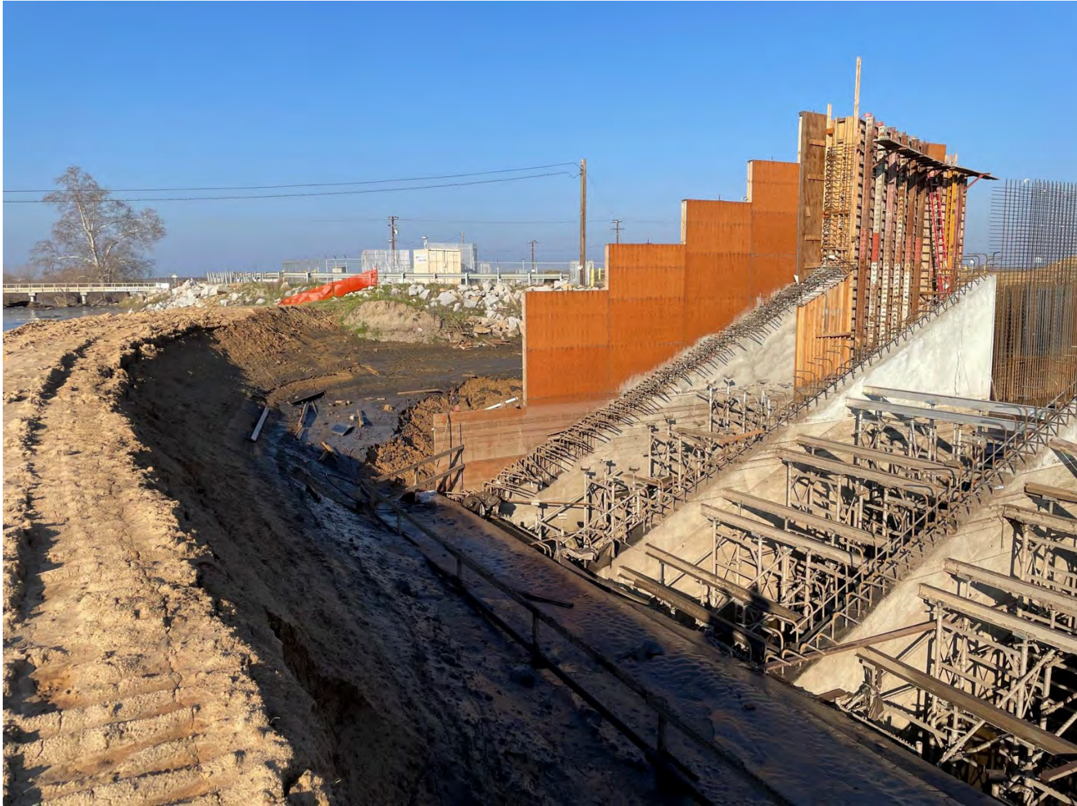
Photo 5: Siphon Structure on North Side of Deer Creek, East of Friant-Kern Canal
