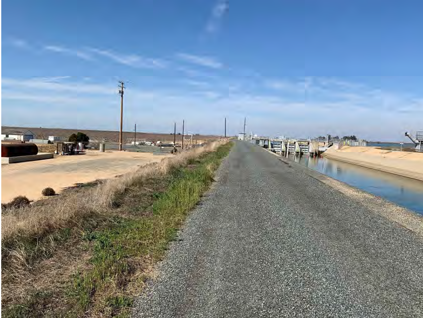
Photo 1: Gravel Improved Access Road Along FKC
