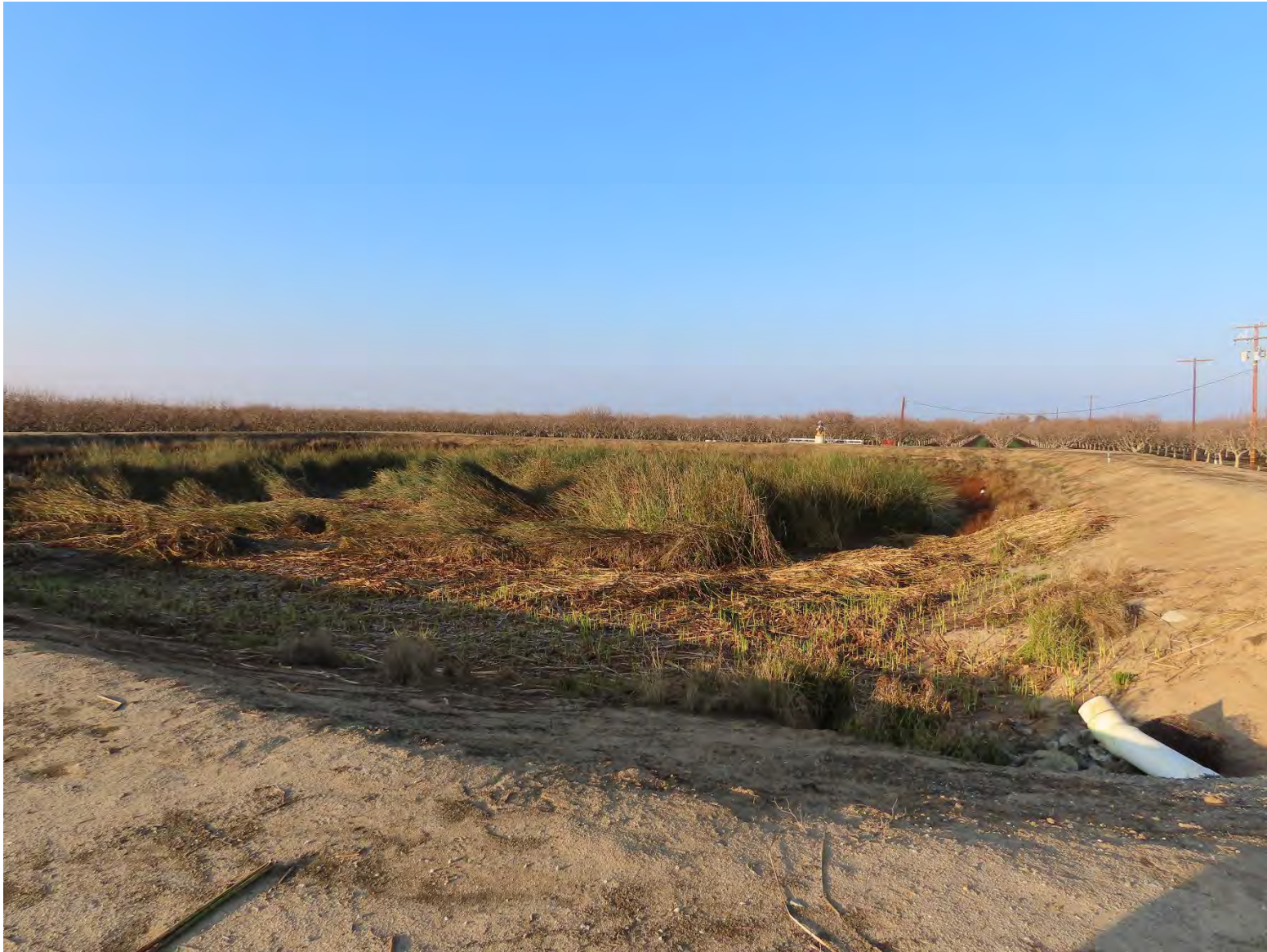
Photo 3: Drained Pond West of the Friant-Kern Canal
