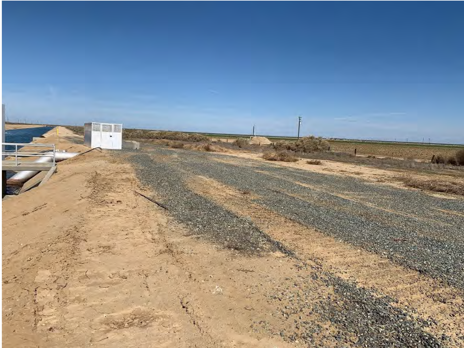
Photo 2: Gravel Improved Access Road
