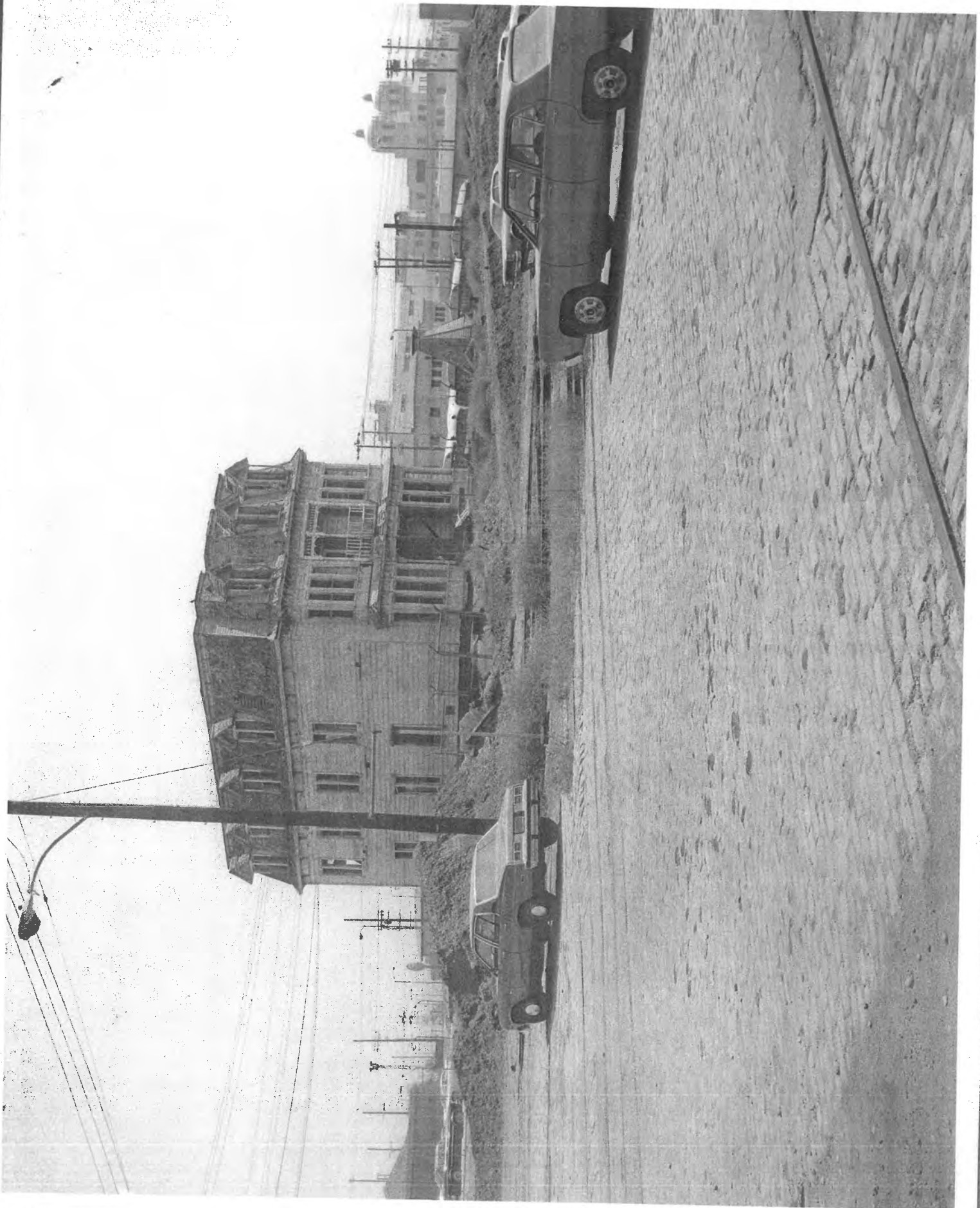
211. GRANITE-BLOCK PAVING, Bruno Street between Alameda and North Main streets. This short, local industrial street, just north of Civic Center and southwest of Chinatown, is unique and historical. The street is the last surviving
