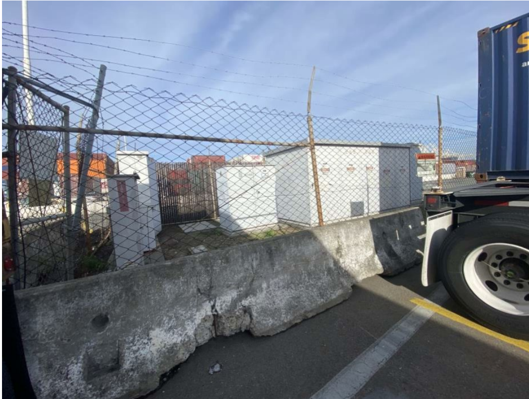
Photo 3.5-1. SS-C-36 Looking West (Montrose Environmental 2023)
