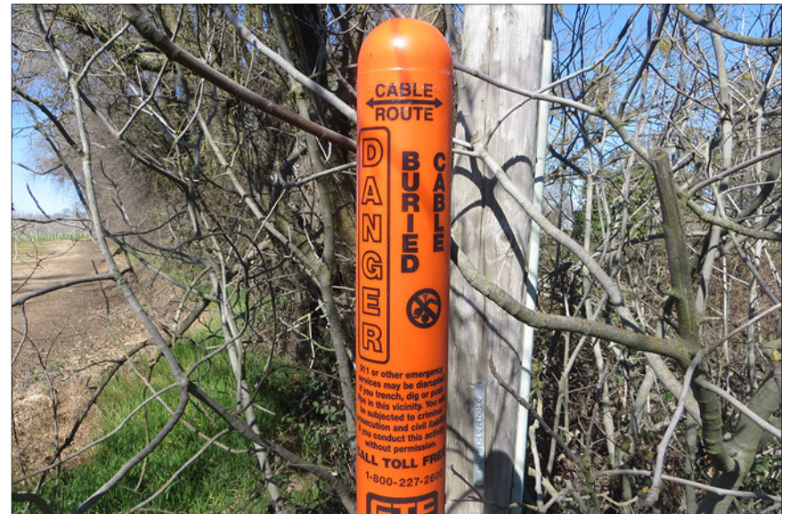
Underground utility marker located in the western terminal of Messick Bridge.
