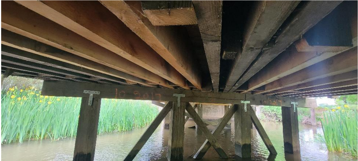
Photograph 5: Standing beneath the bridge over Moshers Creek looking along the underside of the bridge towards the east from the western end.
