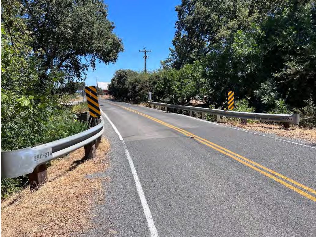
Photograph 1: Northeast-facing view toward Messick Road Bridge.
