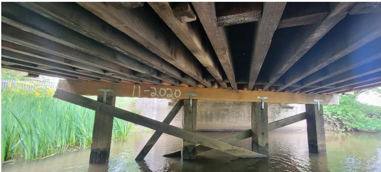
Photograph 6: Standing beneath the bridge over Moshers Creek looking along the underside of the bridge towards the east from the middle of the creek.
