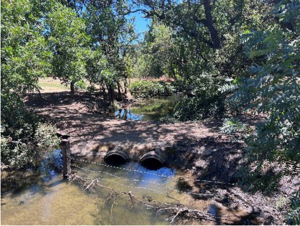
Photograph 1: Standing on the bridge over Moshier Creek looking south along the creek.
