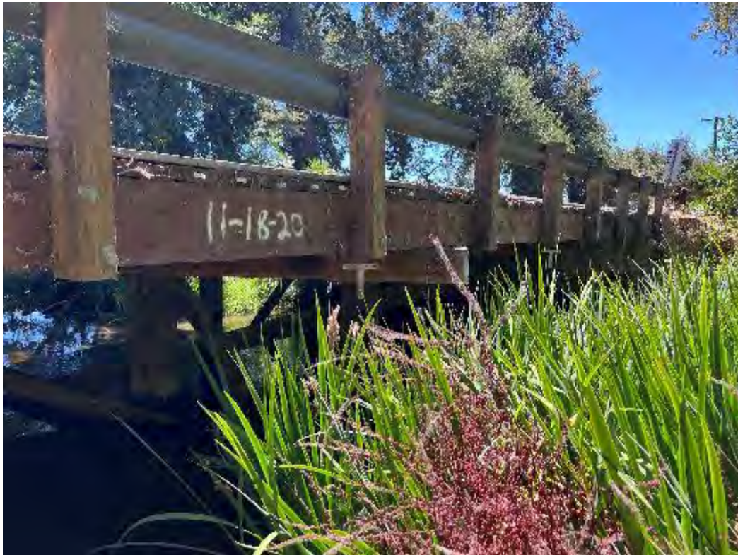
Photograph 6: Standing in Moshier Creek looking west along the north side of the bridge.
