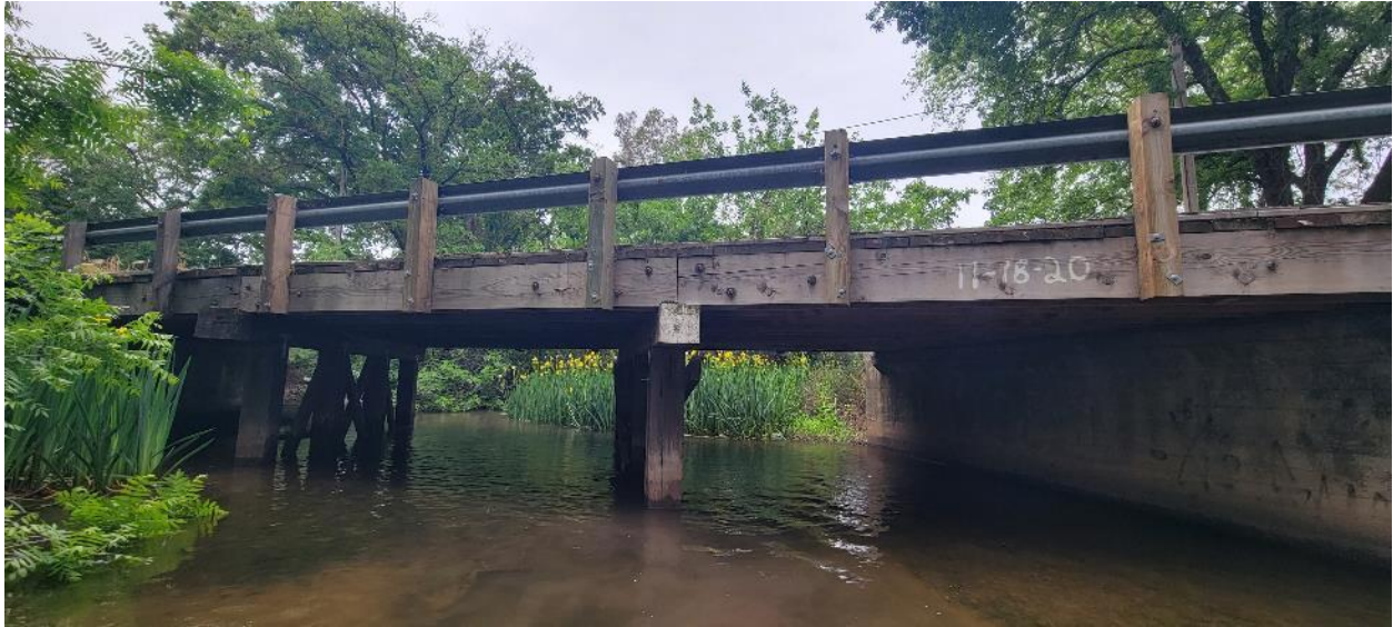
Photograph 1: Standing on the south side of the bridge over Moshers Creek looking north.
