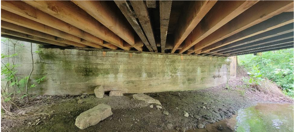
Photograph 3: Standing beneath the bridge over Mosher Creek looking towards the western abutment.
