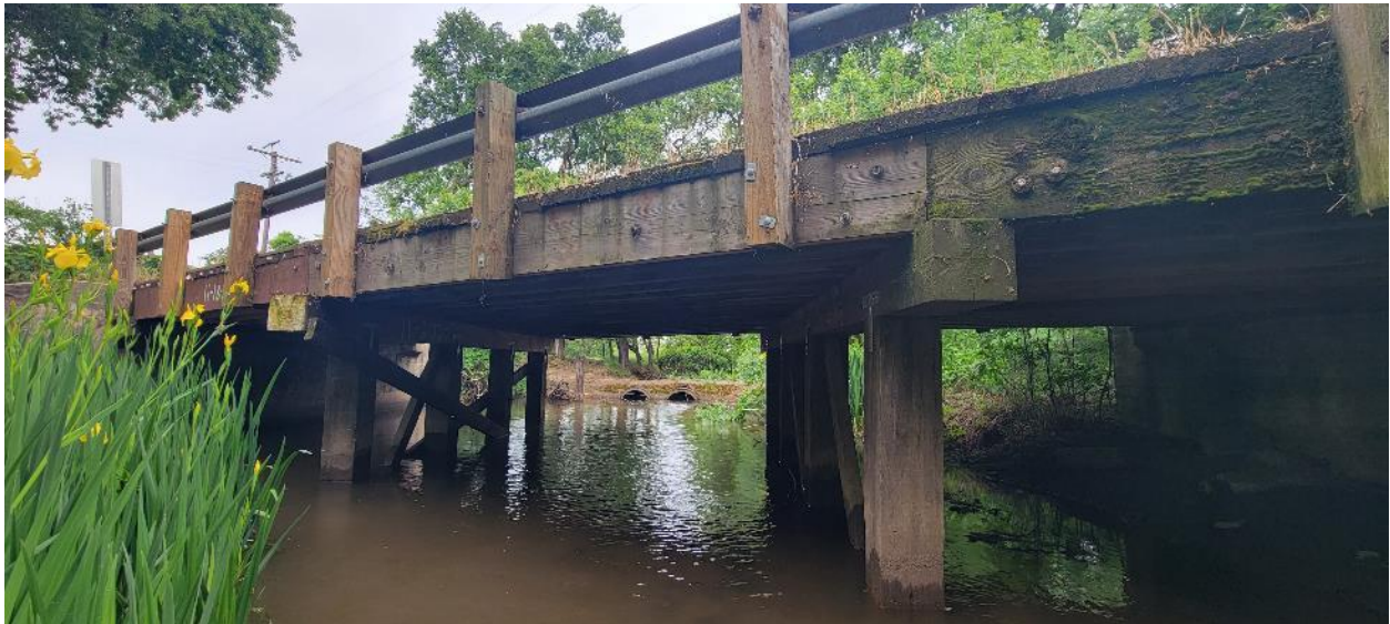
Photograph 2: Standing on the north side of the bridge over Moshers Creek looking south.
