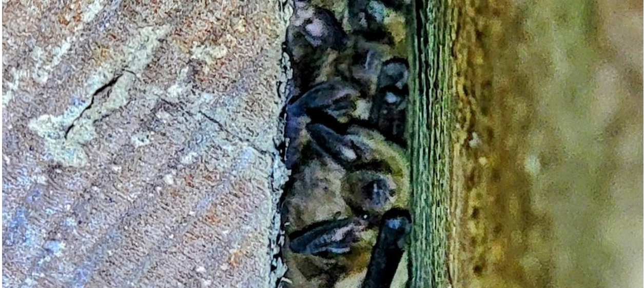
Photograph 7: Yuma myotis observed within a crevice in framing on the underside of the bridge over Mosher Creek.
