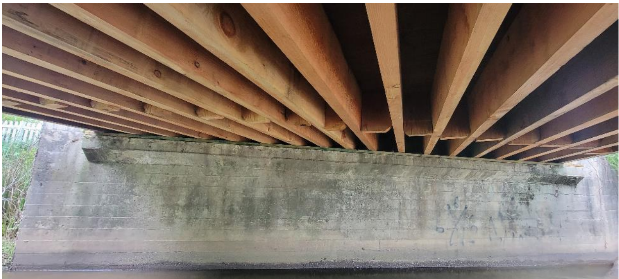
Photograph 4: Standing beneath the bridge over Mosher Creek looking towards the eastern abutment.
