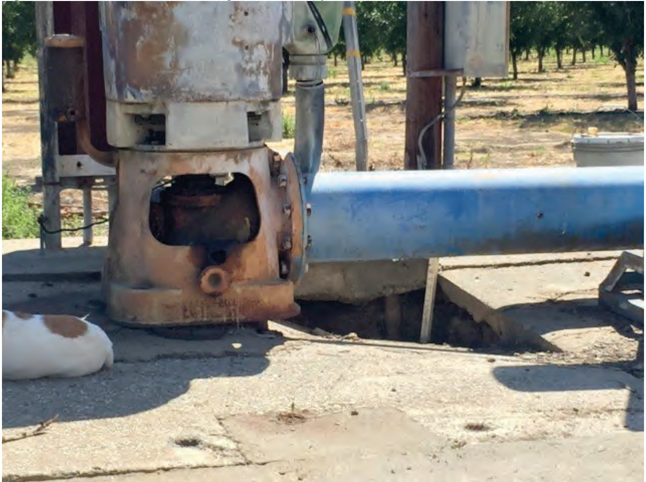
Figure 2. Subsidence on Billiou Well #35 pad. June 2015 (by Billiou).
