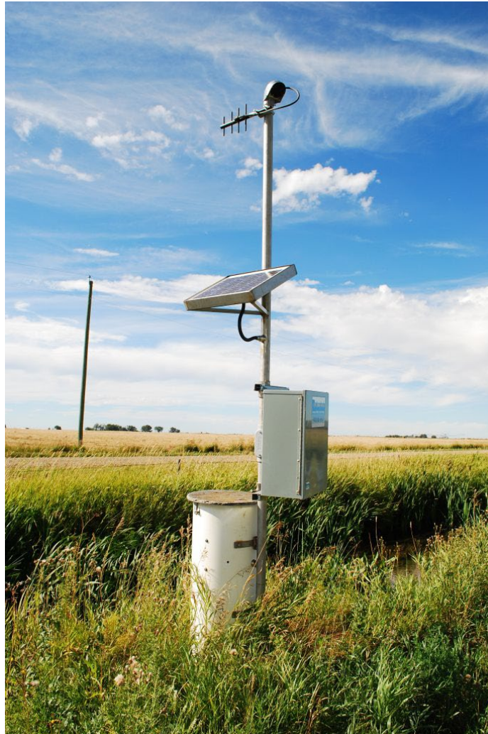
Photograph 1 Wireless SCADA System Example
