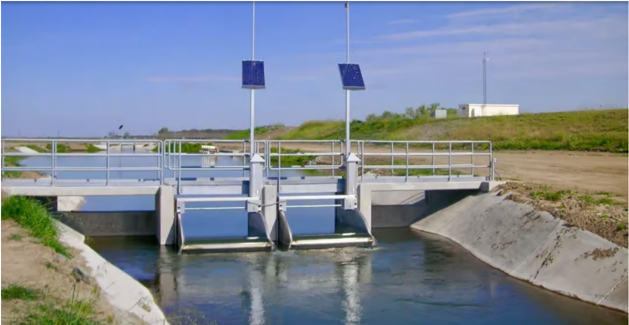
Photograph 2 Automated Gate Installation Example
