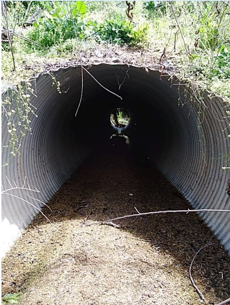
Photograph 7: Outflow culvert to Drainage Segment 1-4. West end of Culvert Segment 1-3.
