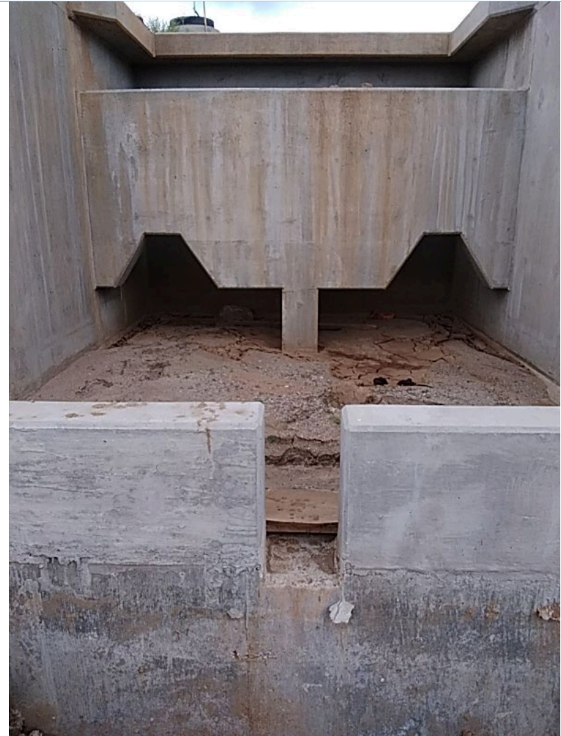
Photograph 6: Cement culvert feeding Drainage Segment 3-1 and floodplain.
