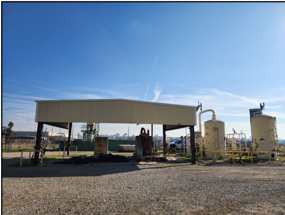
Plate 6: Overview of a steel equipment shelter, facing north.
