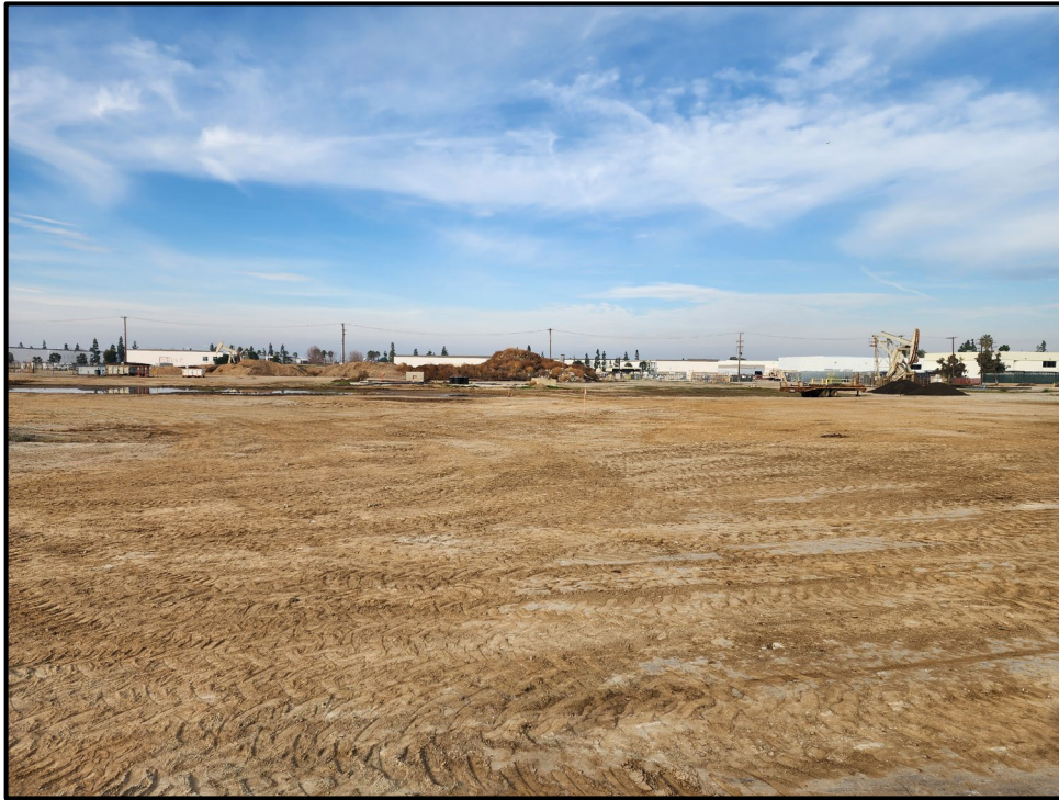
Plate 1: Overview of the subject property, facing south.
