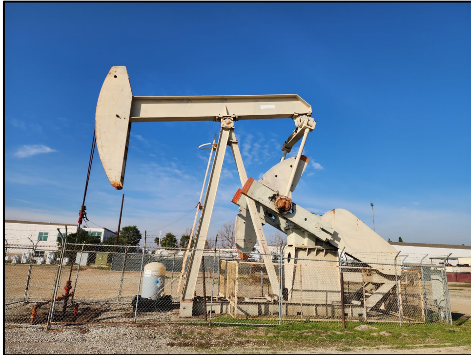
Plate 3: One of six pumpjacks identified on the subject property, facing west.
