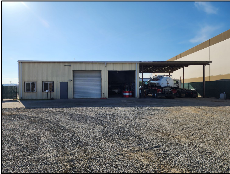
Plate 5: West façade of the main steel building on the property, facing east.
