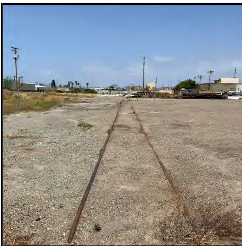
Figure 12. Defunct track existing within previously recorded site boundaries (view north-northwest). May 3, 2022.
