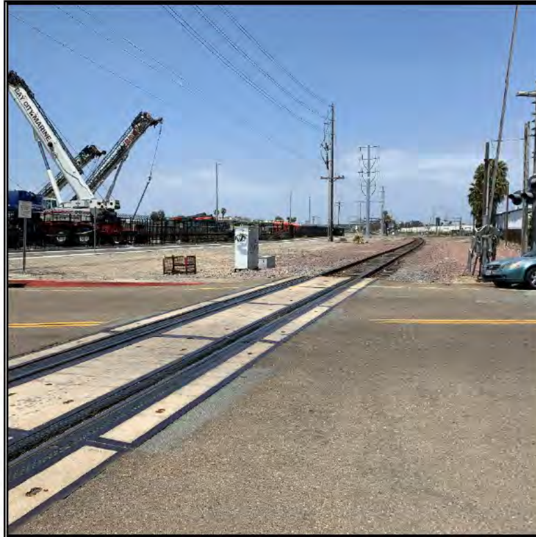
Figure 10. NCD-005 Civic Center Drive (view north). May 3, 2022.
