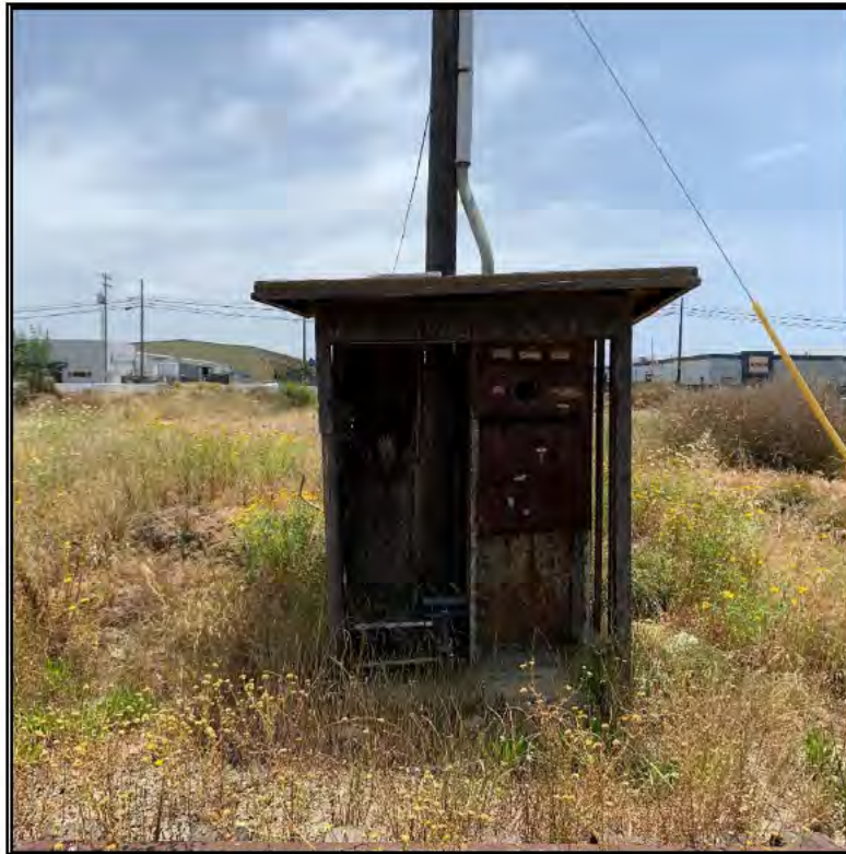
Figure 8. NCD-003 structure (view south). May 3, 2022.
