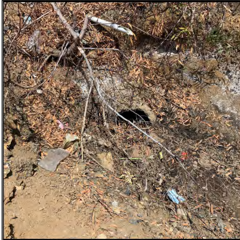
Figure 6. NCD-001 culvert pipe (view east). May 3, 2022.
