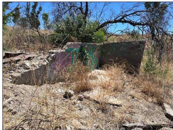
Photo 20. CA-RIV-5075H wall ruins; view east.
