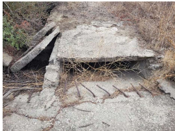
Photo 18. CA-RIV-5073H, showing entrance to drain; view south.
