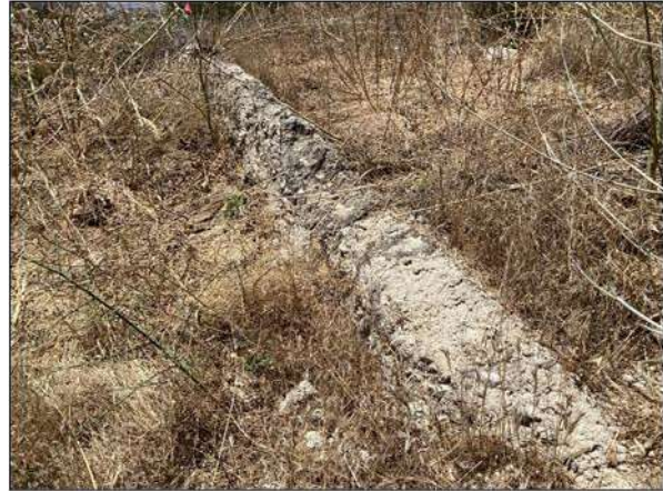
Photo 22. CA-RIV-5075H footing close up.
