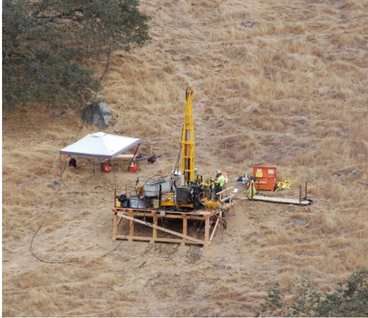
Helicopter-portable Drill Rig on Temporary Platform
