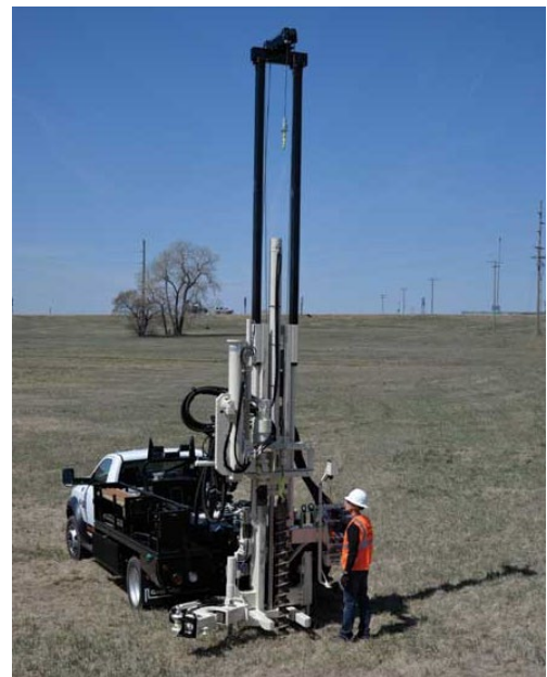
Truck Mounted Drill Rig
