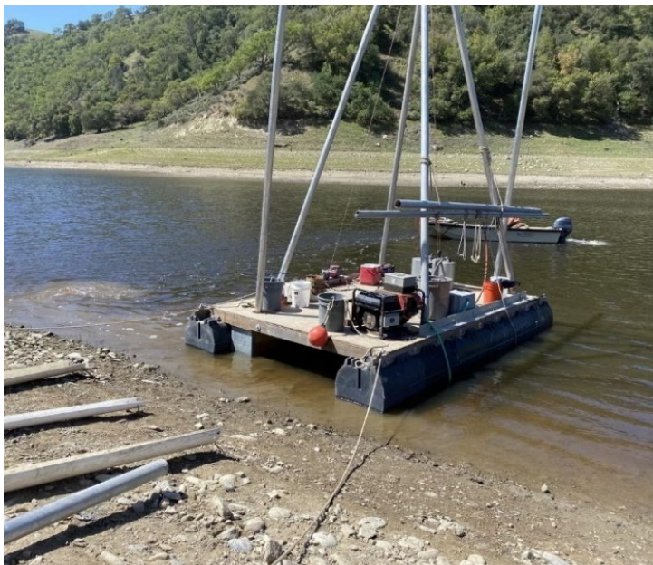
Barge-based Vibracore Drill Set Up
