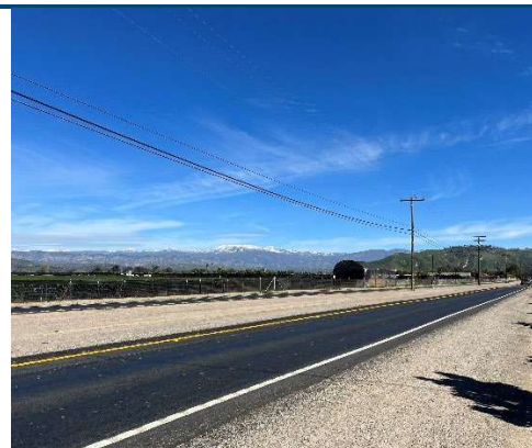
23RW-60 Rose Avenue, Across Oriented N, 4,280 ft from South end of RW
