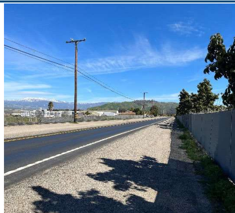
23RW-70 Rose Avenue, 5,290 ft from South end of RW
