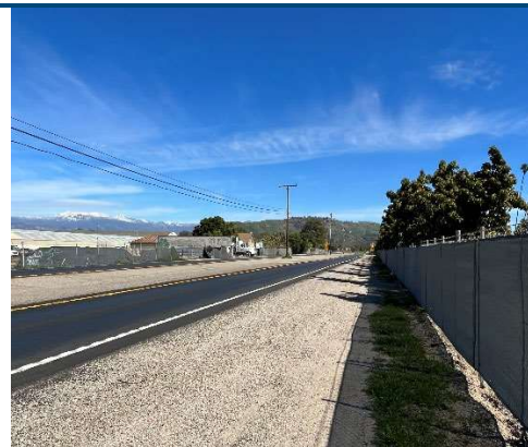
23RW-72 Rose Avenue, 5,710 ft from South end of RW
