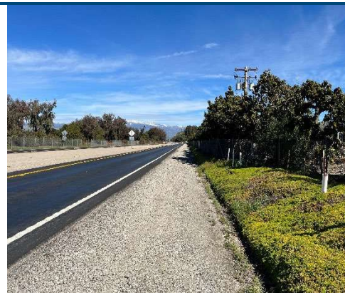
23RW-84 Rose Avenue, 6,880 ft from South end of RW
