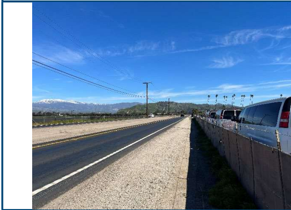
23RW-57 Rose Avenue, 3,645 ft from South end of RW
