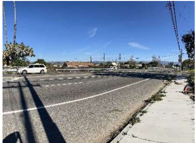
21RW-02 Rose Avenue, Across Oriented NW, 40 ft South of ROW Acquisition area
