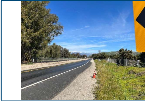
23RW-81 Rose Avenue, Across Oriented N, 6,660 ft from South end of RW
