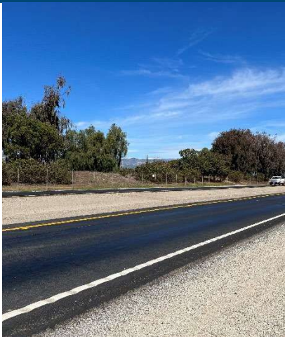
23RW-89 Rose Avenue, Oriented N, 7,500 ft from South end of RW
