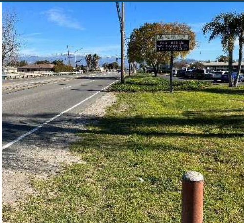
23RW-03 Rose Avenue, 180 ft from South end of ROW Acquisition area
