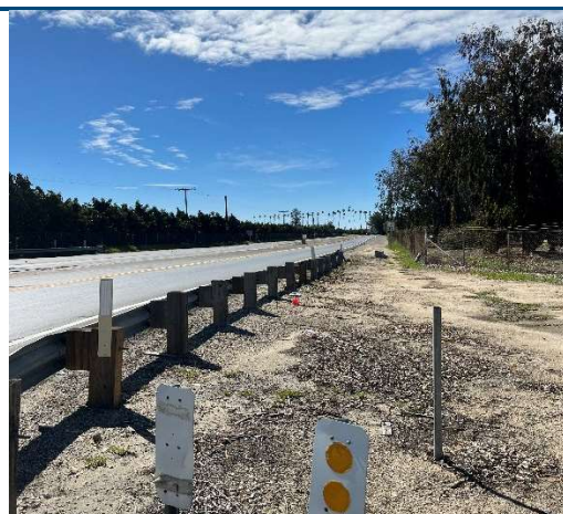
23RW-98 Rose Avenue, Oriented NW, 8,050 ft from South end of RW, South bound shoulder (Rose Ave and Hwy 118 Intersection)
