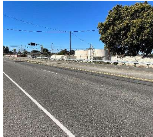
23RW-20 Rose Avenue, Across, Oriented SW 1,300 ft from South end of ROW Acquisition area
