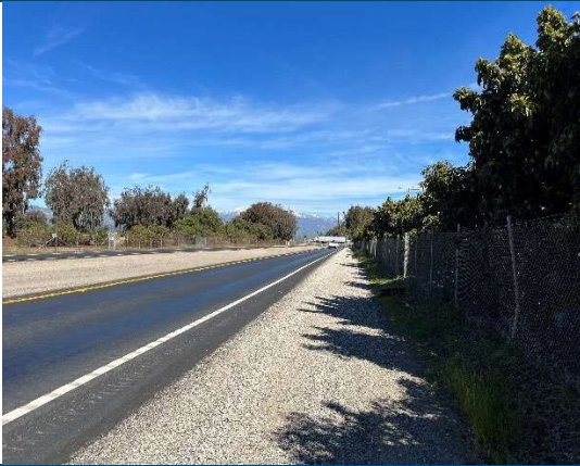
23RW-87 Rose Avenue, 7,240 ft from South end of RW
