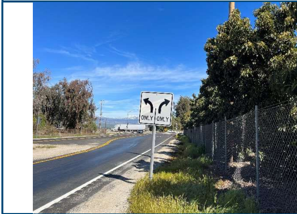
23RW-93 Rose Avenue, 7,730 ft from South end of RW
