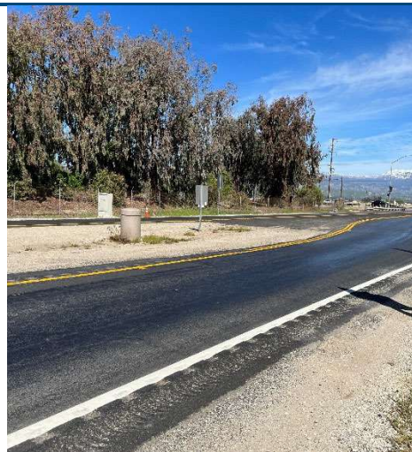
23RW-92 Rose Avenue, Across Oriented N, 7,730 ft from South end of RW
