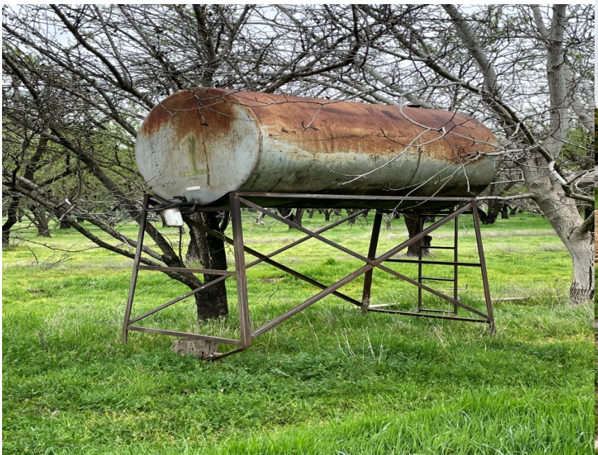
Photo 3: View of empty decommissioned AST
