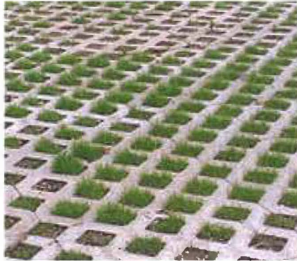
Using green infrastructure and features such as permeable pavers reduces impacts on the environment.
