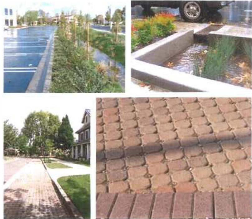
Green infrastructure can include features such as swales, vegetated buffers, sand filters, and artificial wetlands, which can be used to manage stormwater runoff and improve stormwater quality. Permeable paving reduces stormwater runoff and produces smaller increases in ambient air temperature than more energy-absorptive traditional paving materials
