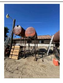
550-gallon and 350-gallon diesel aboveground storage tanks
