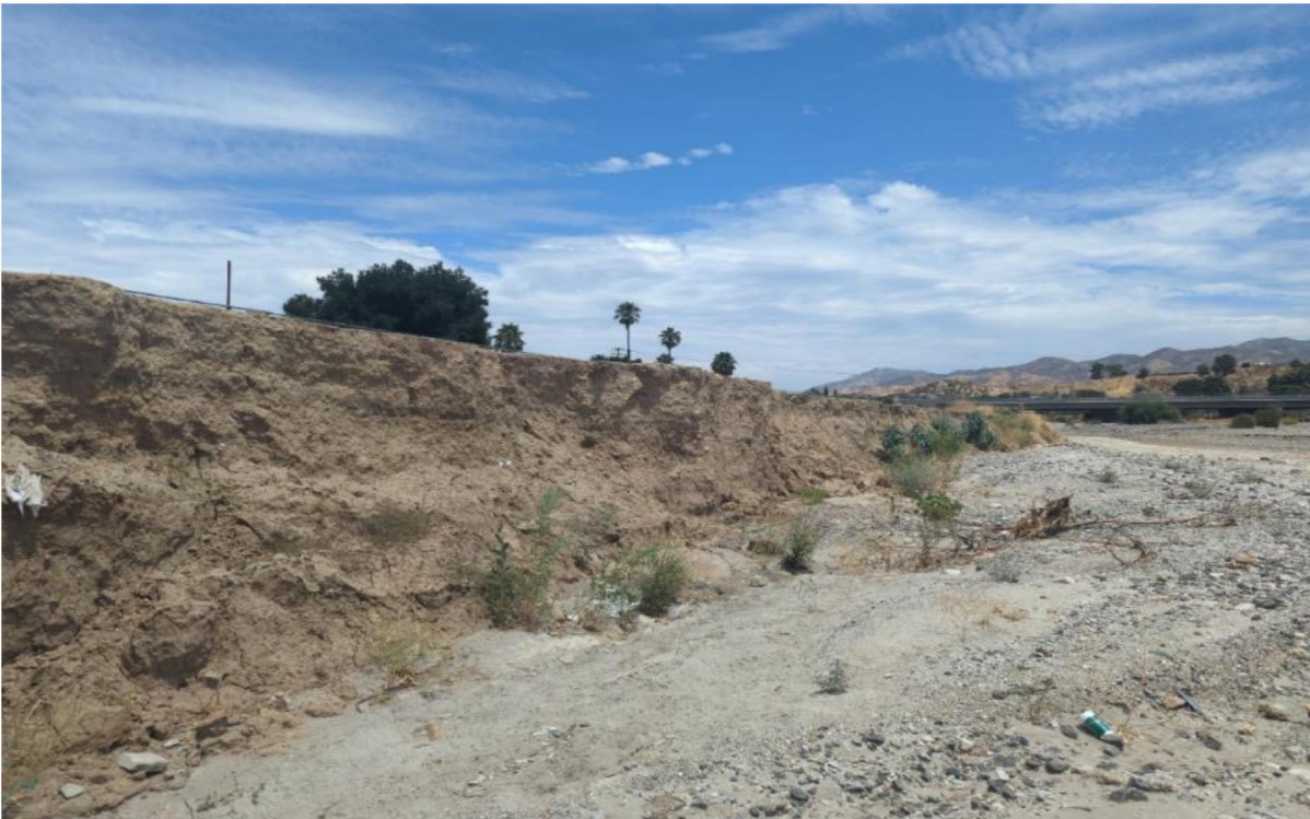
Photograph 18. Photo Point 18. View of the northern bank of the SCR in the central portion of the APE where soil cement bank protection is proposed, facing east. Note unstable, eroding bank (August 1, 2023).
