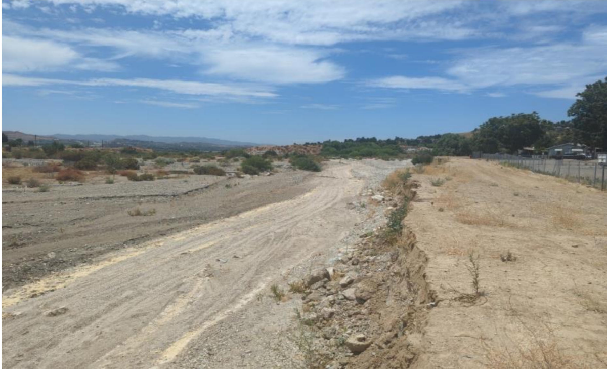
Photograph 15. Photo Point 15. View of the northern bank of the SCR in the central portion of the APE where soil cement bank protection is proposed, facing west. Note unstable, eroding bank and compacted, barren soils immediately north of the bank (August 1, 2023).
