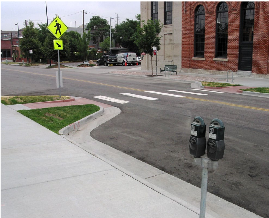
A pinch point is a horizontal extension of the curb at a midblock point of a street resulting in a narrower roadway.
