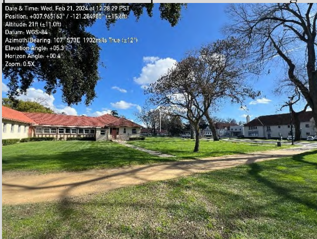
Photo 9. View facing southeast toward Building 2 pictured left.
