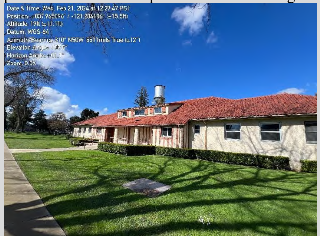
Photo 10. View facing northeast toward Building 2.
