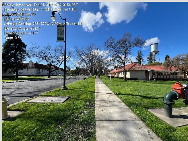
Photo 12. View facing west toward Building 1 pictured left and Building 2 pictured right.
