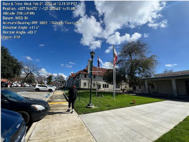
Photo 1. View facing southeast at Building 1.
