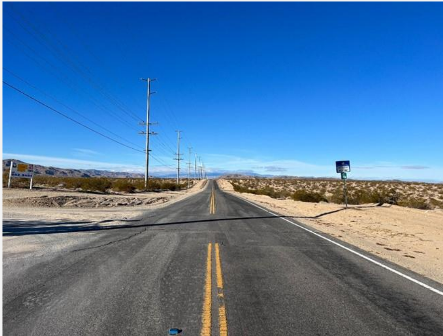
Exhibit 3. Overview of asphalt-paved Two Mile Road, view facing west
