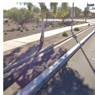
Bike separation option A (18" Concrete header)
