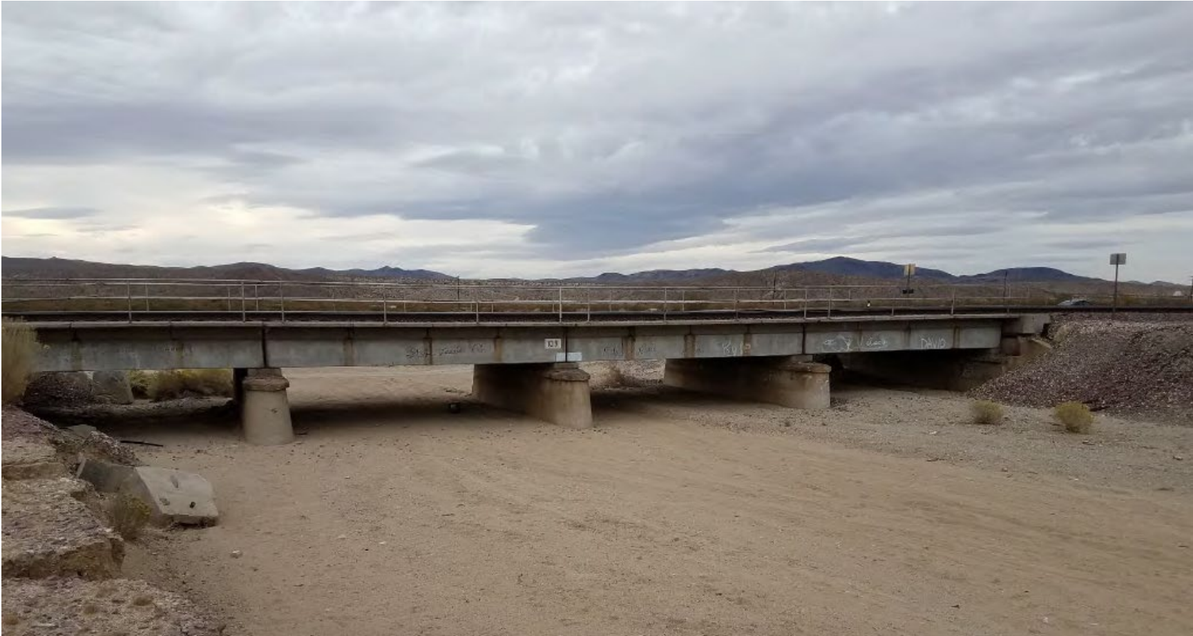
Figure 7: Existing Mainline Bridge 10.9
