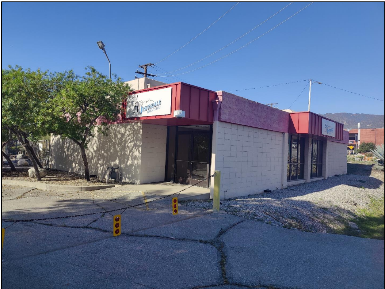
Figure 17. Training Center, south façade (left) and east elevation (right), facing northwest.
