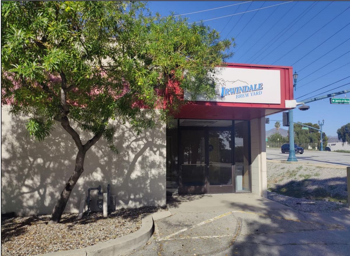
Primary entrance at south façade, facing north.
