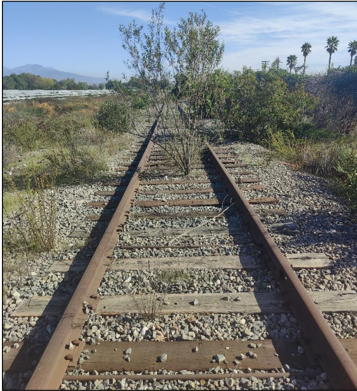
West/east segment of AT&SF spur, facing east.
