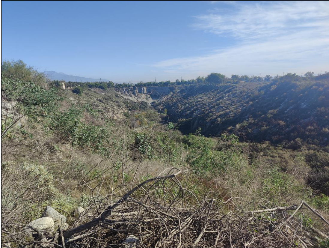
Overview of quarry from westernmost end, facing east.
