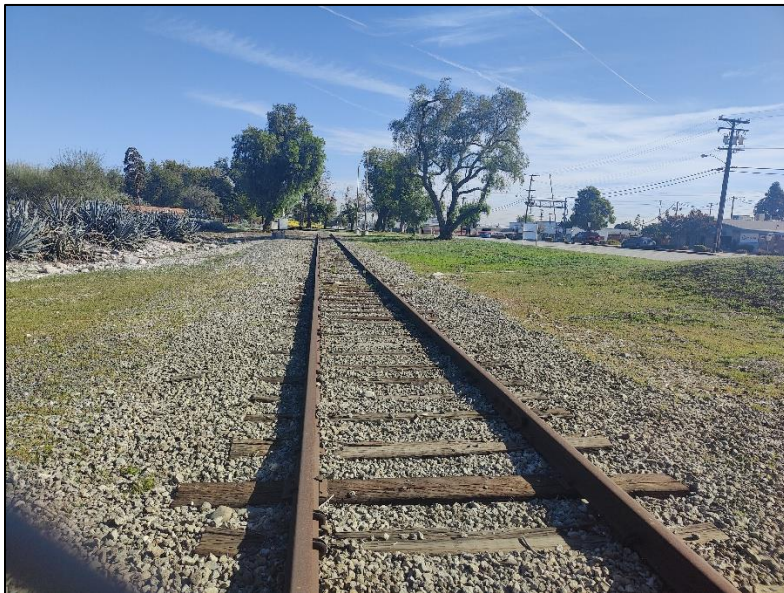
Segment of AT&SF connecting with Union Pacific Azusa Industrial Lead at northwest corner of W. 1 st Street and Irwindale Avenue, facing east.
