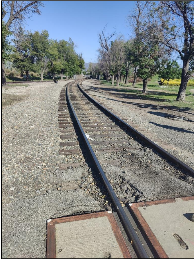
Segment of railroad, facing northeast from West 1 st Street.
