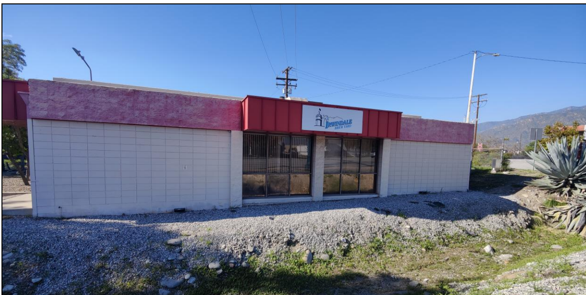
East elevation, facing west.
