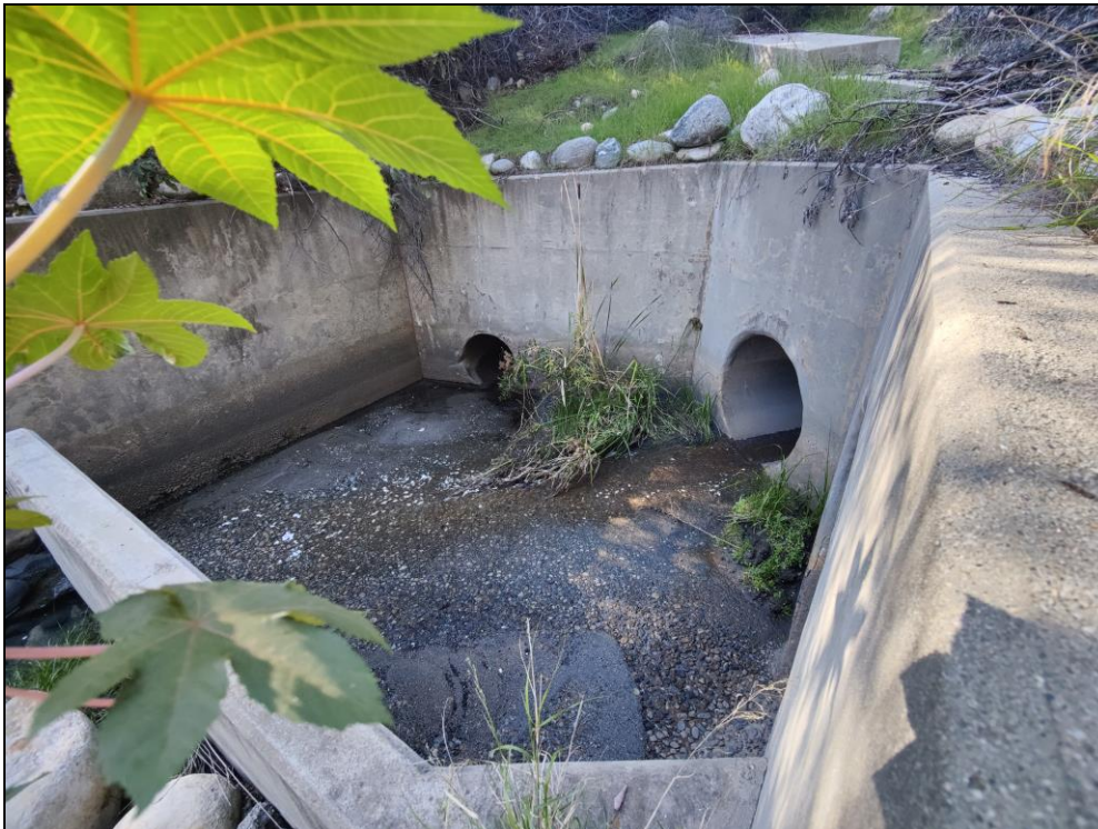
Drainage culvert installed ca. 1990s from MillerCoors brewery to the north, at western end of quarry.
