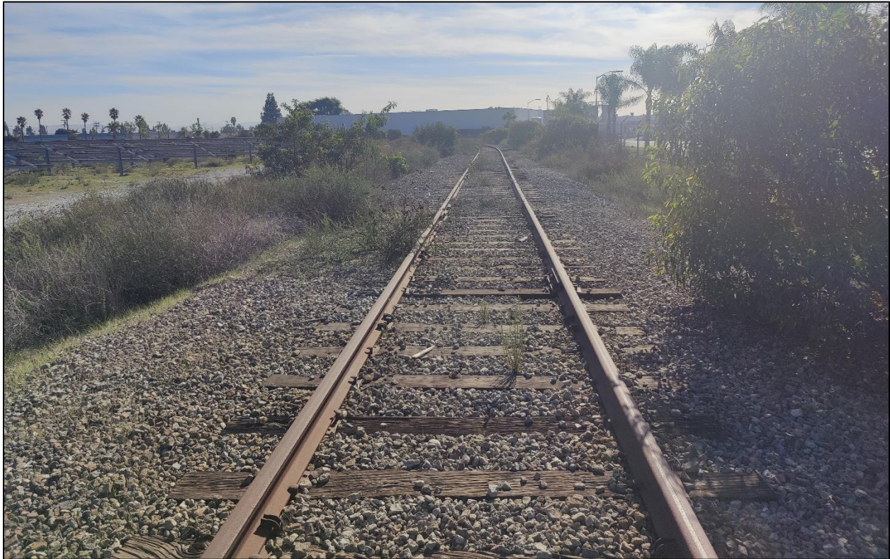
North/south segment of AT&SF spur, facing south.
