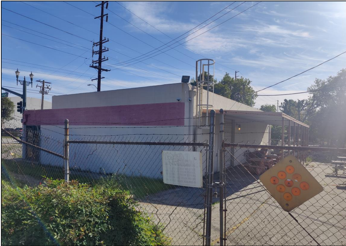
North elevation (left) and west elevation (right), facing southeast.
