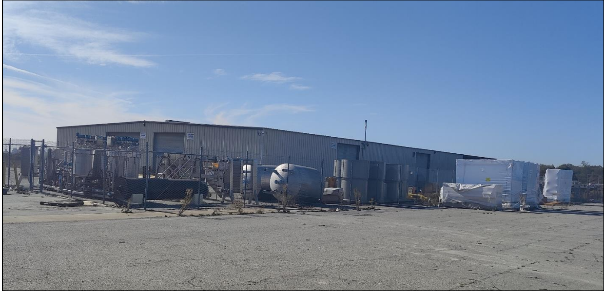
Figure 18. Warehouse, east façade (left) and north elevation (right), facing southwest.
