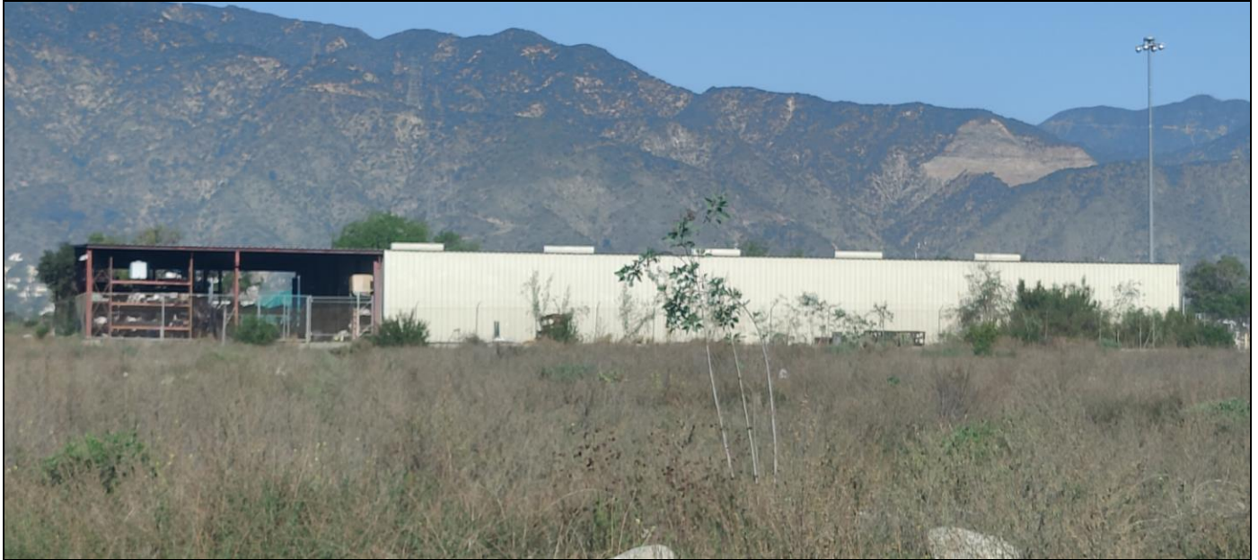
South elevation, facing north.
