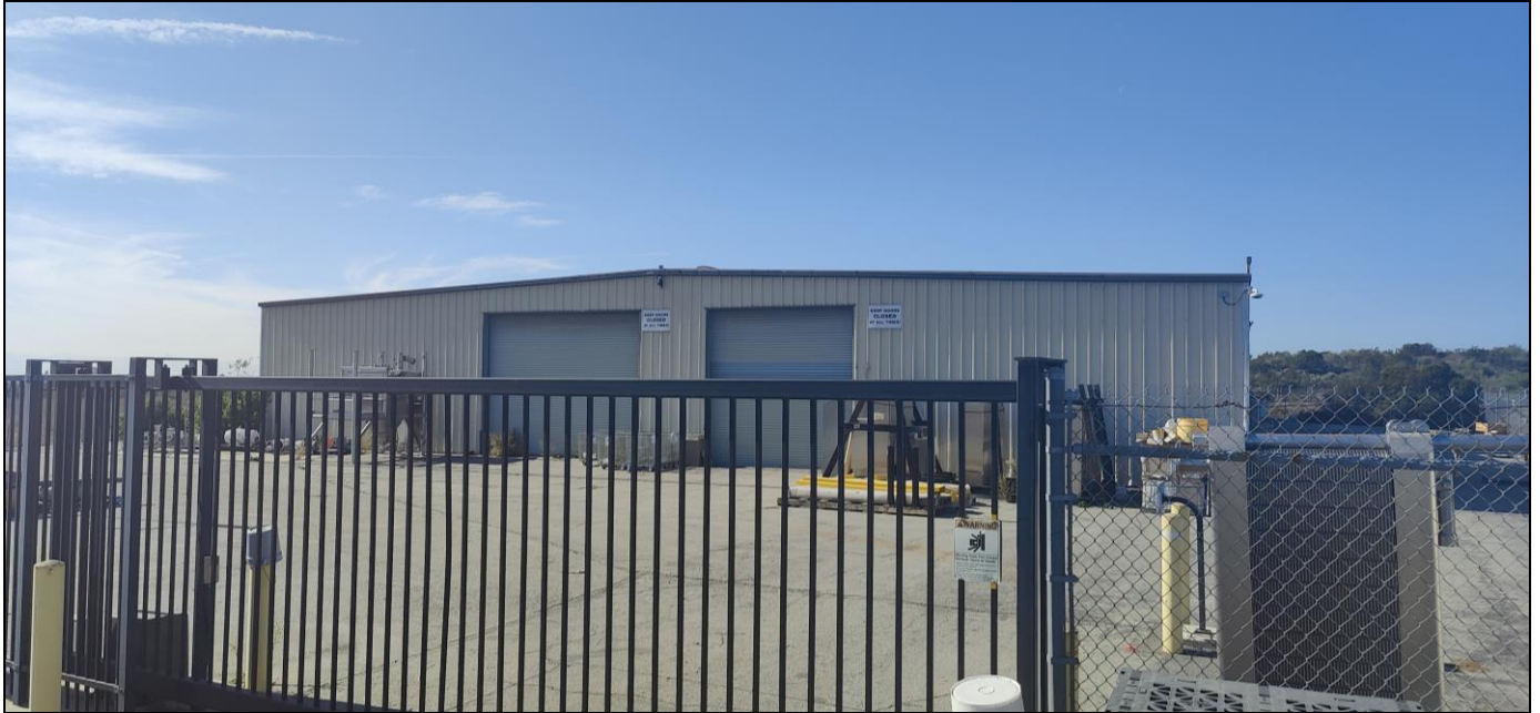
West façade, facing southwest.
