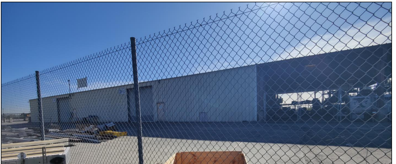
North elevation and partial west elevation, facing southeast.
