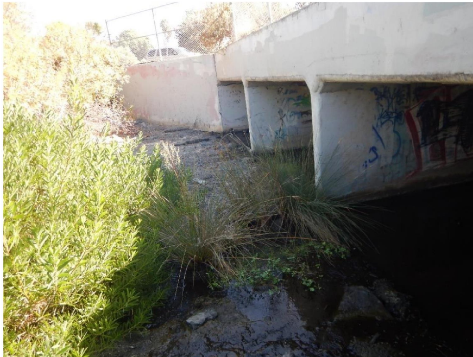
Photo 14: Armoring at downstream end of domain of analysis
