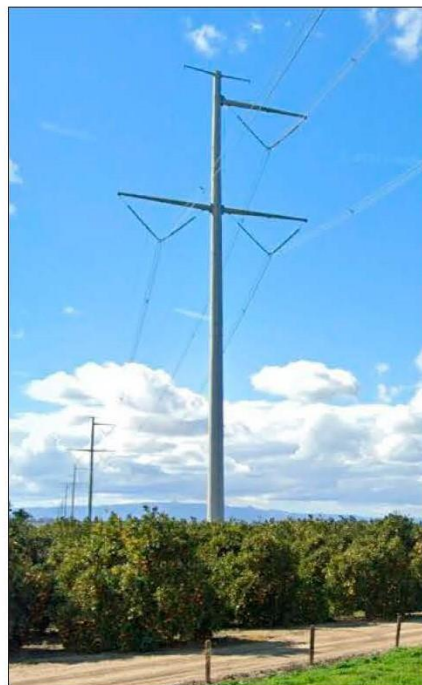
500-kV Single Circuit Monopole - Up to 190 feet
