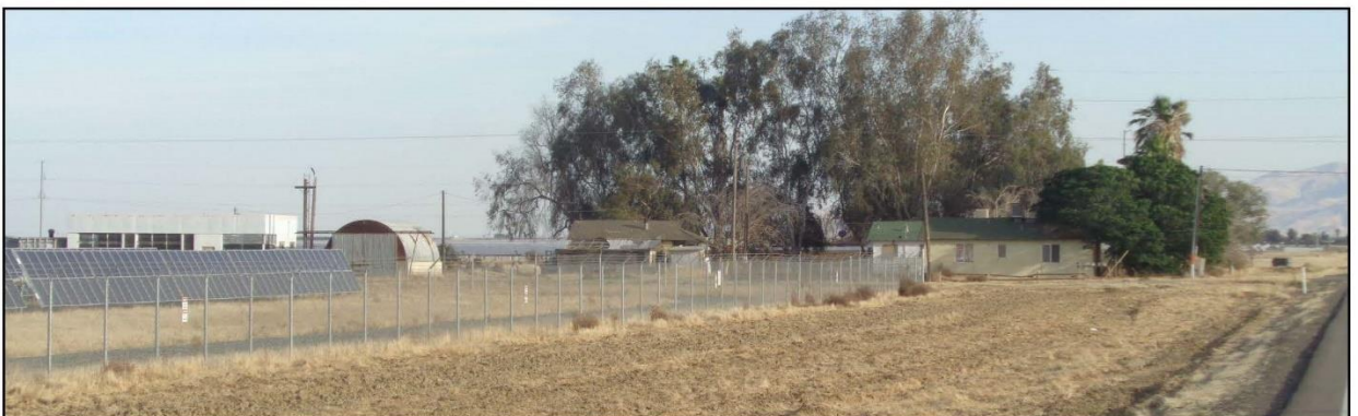
Photo 9: Solar Array with Adjacent Residence
