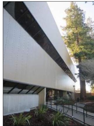
Figure 19. Stepped profile viewed at the north façade, formed by outward-angled windows at the first and second floors
