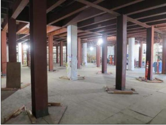
Figure 14. Basement-level open space at the west end of SC1, containing non-original structural supports
