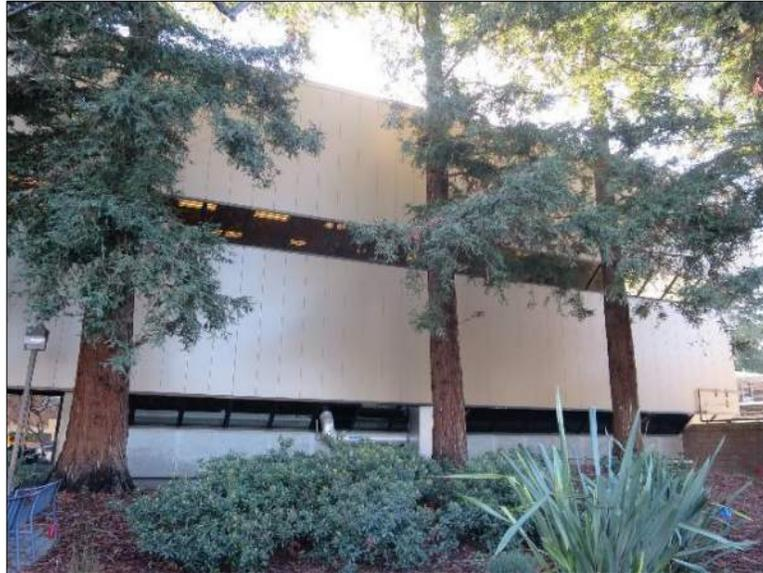
Figure 12. SC2's typical exterior configuration of window bands separating broad, opaque areas of metal panel cladding, viewed at the north façade
