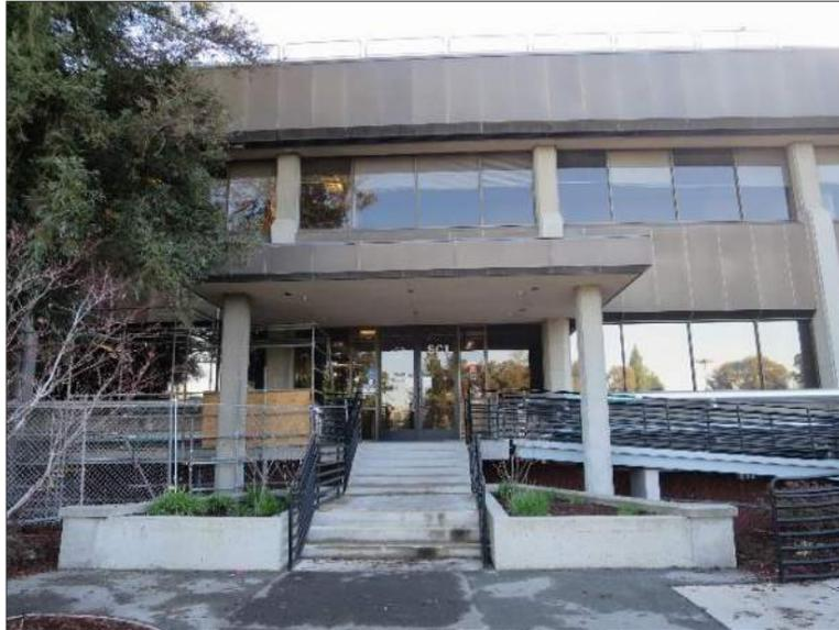
Figure 6. Entrance centered on the north façade, featuring concrete landing, canopy, steps, ADA ramp, and planting beds
