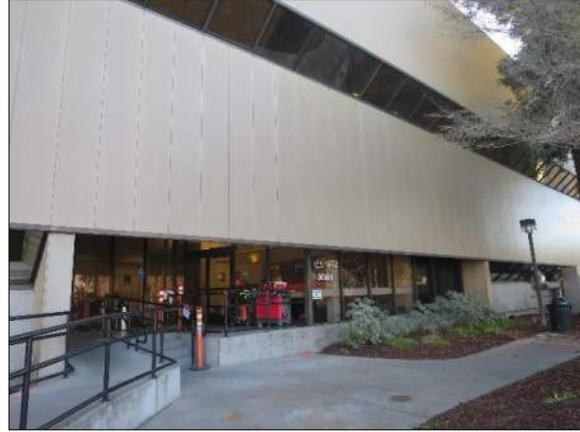
Figure 21. First-floor entrance at the center of the north façade, featuring a recessed vestibule with concrete landing, steps, and ADA ramp
