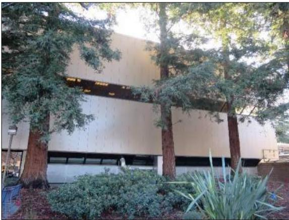
Figure 18. SC2's typical exterior configuration of window bands separating broad, opaque areas of metal panel cladding, viewed at the north façade
