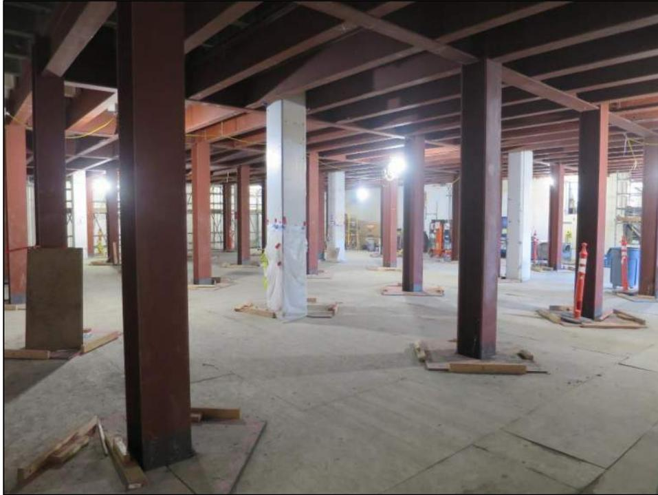
Open space with steel structural columns in the basement level of SC1
