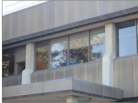
Figure 5. Typical grouping of four panes between pilasters, which contribute to the window ribbons that span each façade
