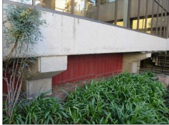
Figure 29. Shaped concrete columns at the basement level of the hyphen, which mimic the appearance of SC1's columns
