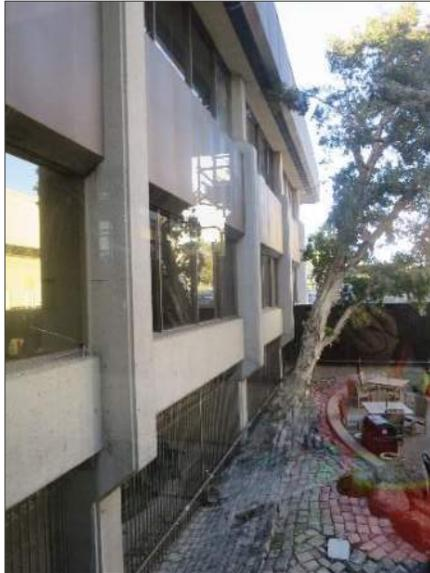
Figure 4. Façade arrangement of pilasters, base, spandrel, and frieze, viewed in profile at the east façade
