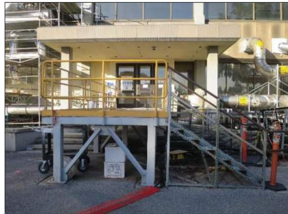
Figure 11. Entrance at the center of the south façade, featuring original canopy and non-original doors and metal gangway
