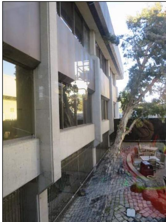
View of the east façade, showing the shaped concrete pilasters and tiered façade configuration
