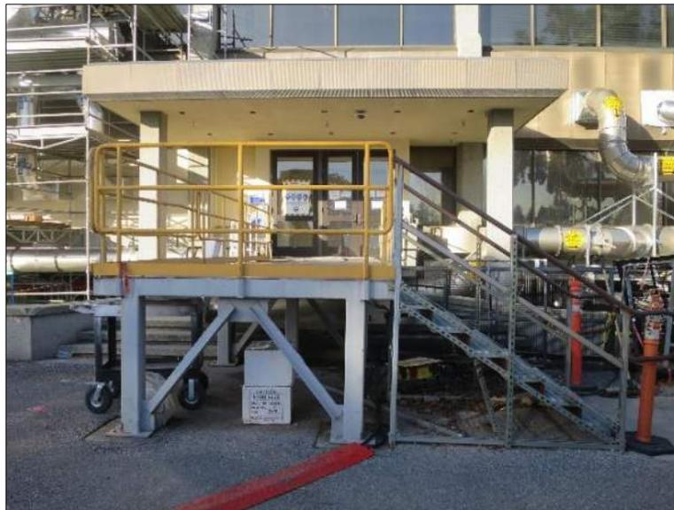
Figure 9. Entrance at the center of the south façade, featuring original canopy and non-original doors and metal gangway
