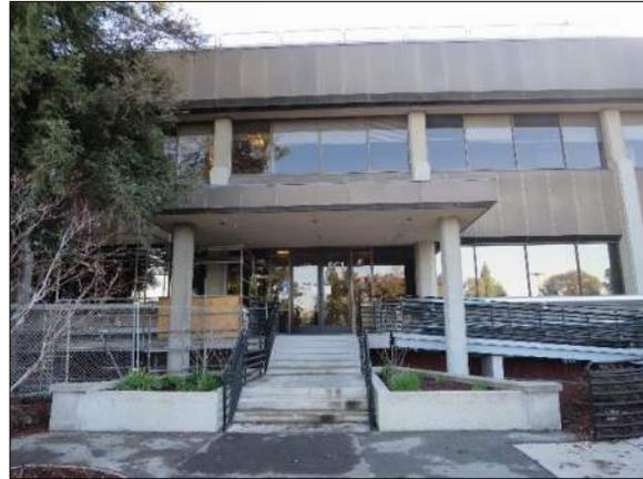
Figure 7. Entrance centered on the north façade, featuring concrete landing, canopy, steps, ADA ramp, and planting beds
