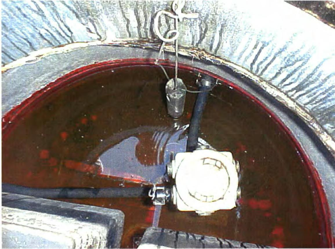
A close up of fill sump shows the sensor tied up and dangling above the water.
