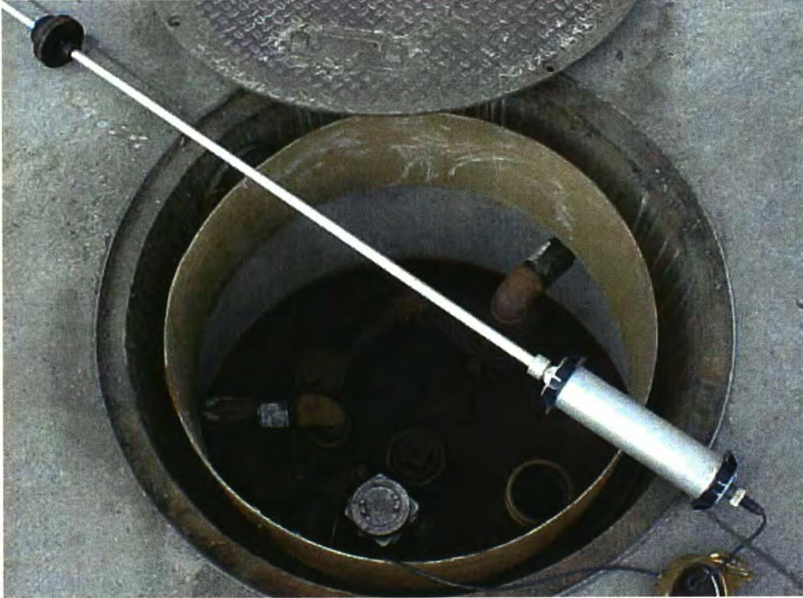
Picture of UST pipe sump. ATG is lying across the top for testing of overfill alarm. The double walled Ameron piping (far left) is covered by a rubber caulder.
