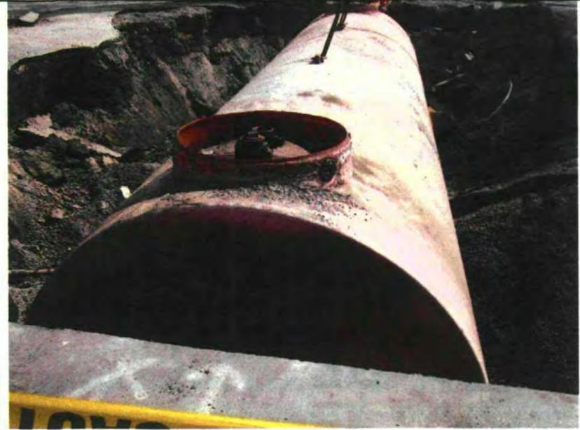
20,000 gallon, glass-steel tank 13 feet in diameter and 38 feet in length. In good condition -no holes noted.
