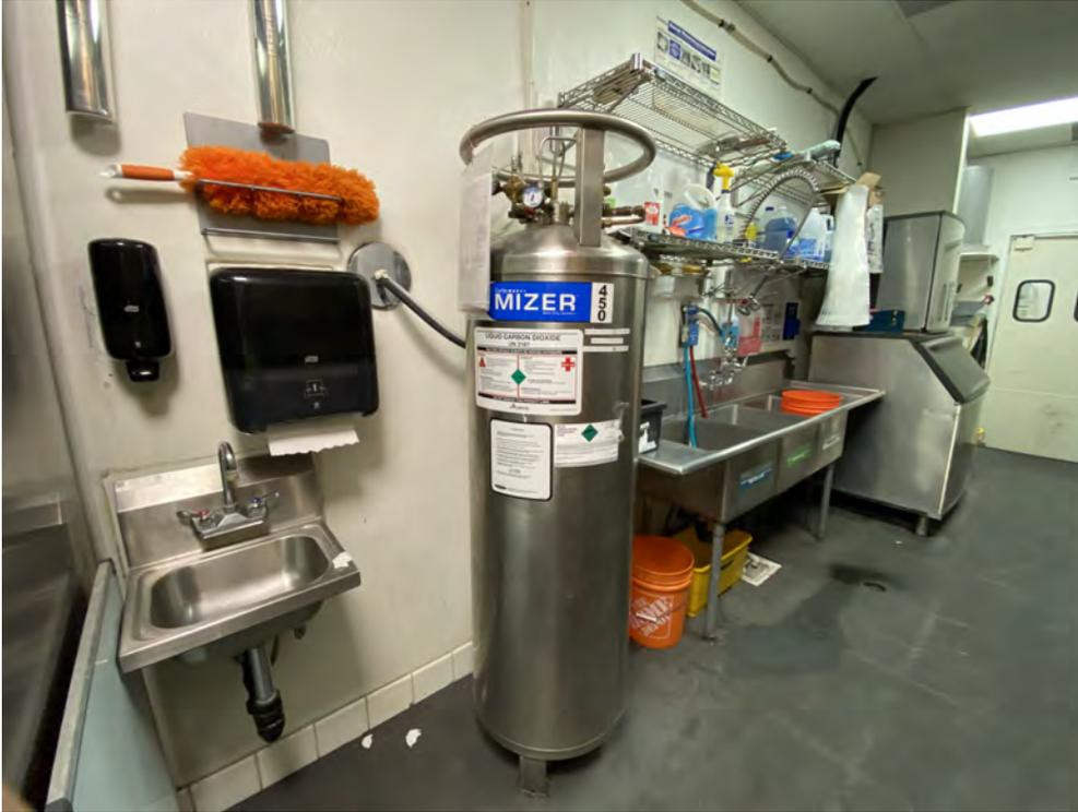
5) A liquid carbon dioxide dewar for beverage carbonation, about 6 feet tall.
