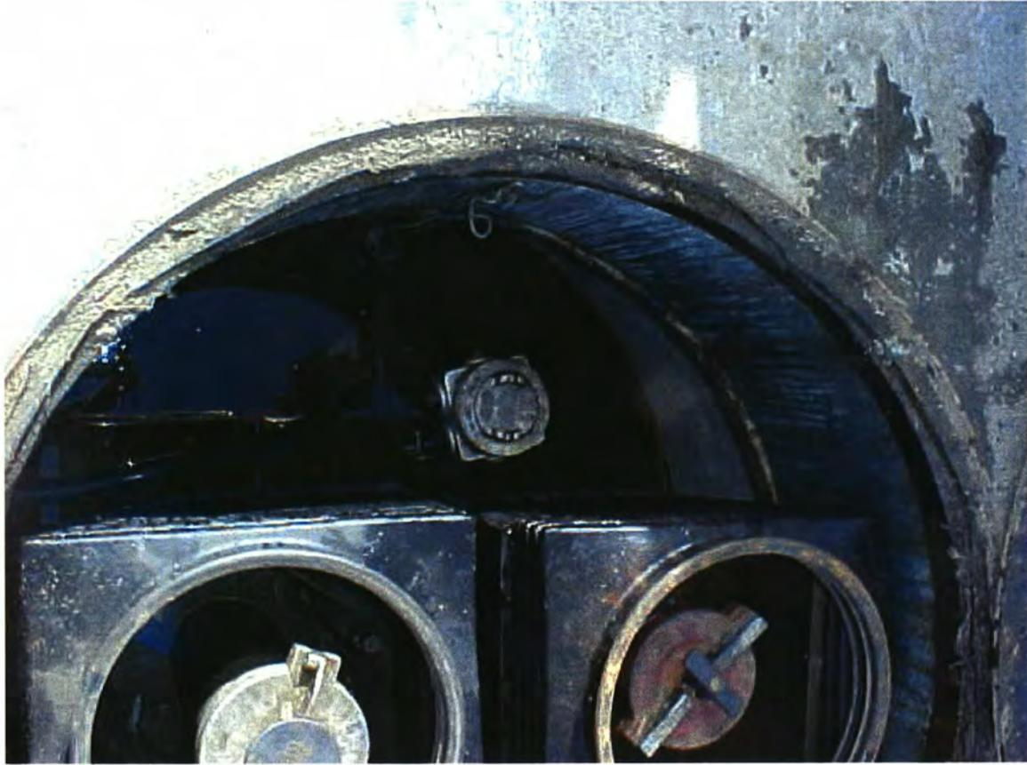
Another view of fill sump, liquid and tampered sensor.
