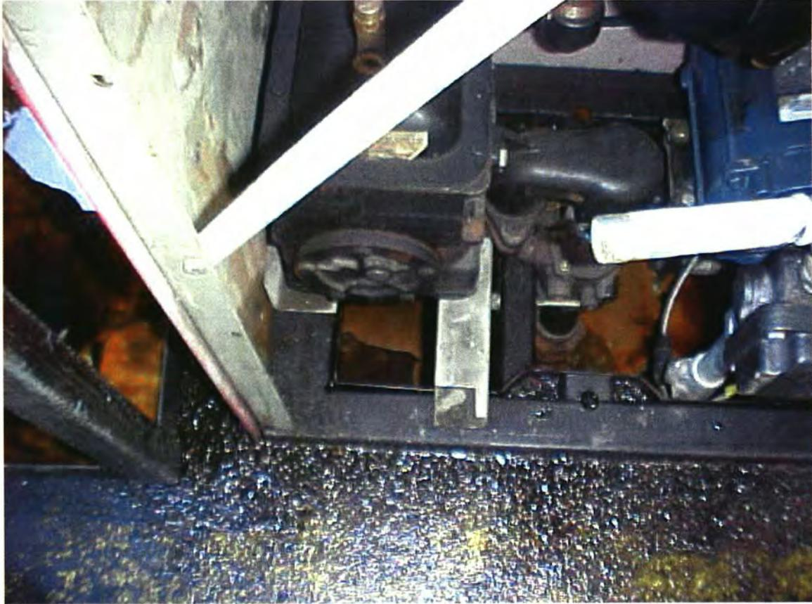
Upon opening the north dispenser (#1), several inches of oil and water were observed. The alarm did not go off because the sensor was tampered with and was dangling above the water.
