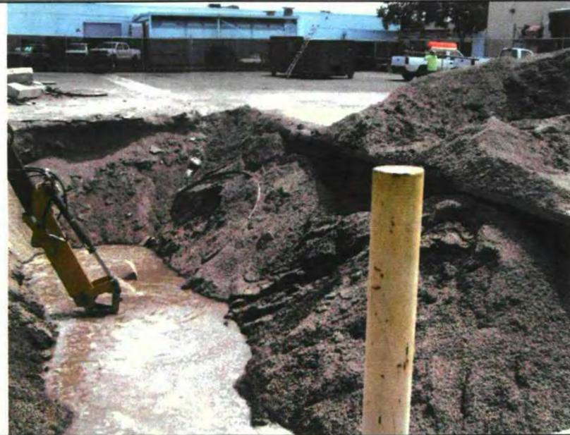
The large amount of pea gravel inhibited the collection of a sample of native material from the east side of the excavation.
