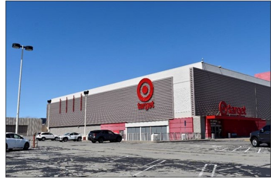
Figure 8. East anchor. Target's south elevation, facing northwest. Source: ICF 2023.
