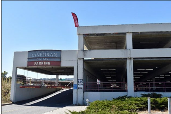
Figure 18. Parking structure #1's entrance from Huntington Avenue, facing southwest.
