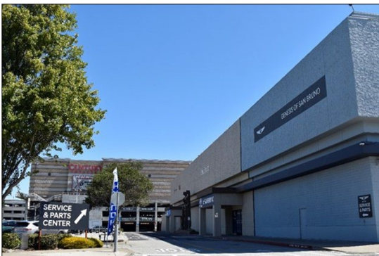
Figure 9. North anchor. Gensis/Hyundai's north elevation, facing east.
