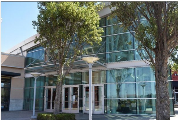
Figure 6. Southwest entrance, facing south. Source: ICF 2023.
