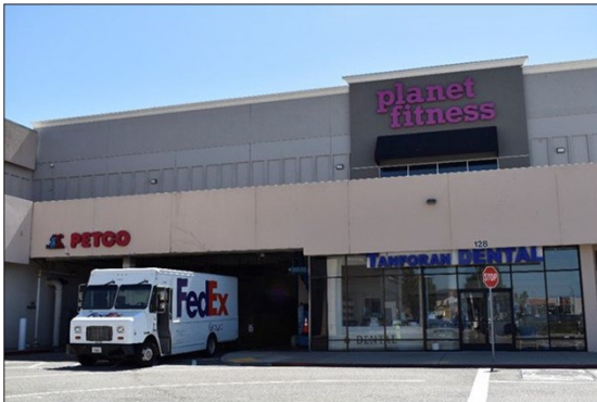
Figure 12. Example of exterior-facing stores' corporate branding. Split ground level. Planet Fitness' north elevation, facing south.
