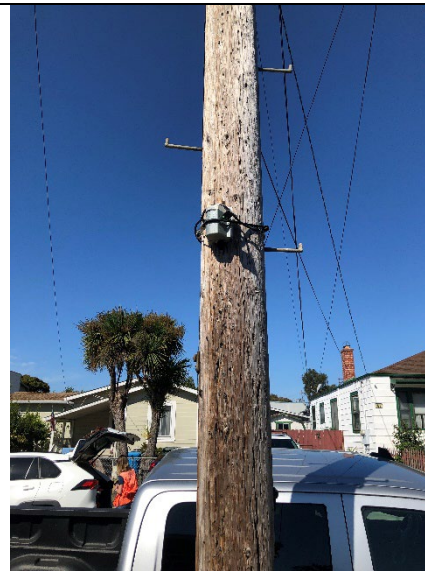
LT-5 Looking Southwest
