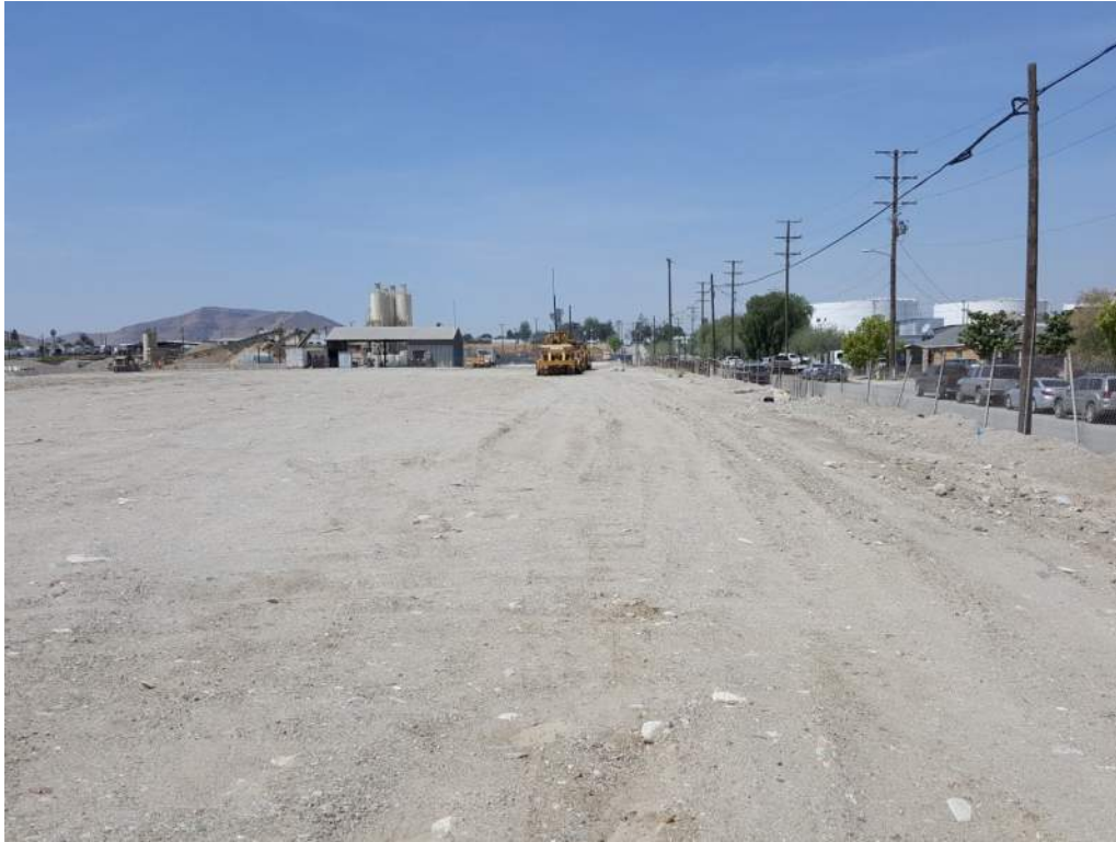
Figure 2. Overview along Santa Ana Avenue, view toward west.
