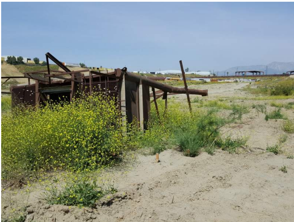
Figure 5. Gravel sorting equipment in basin, view toward northwest.
