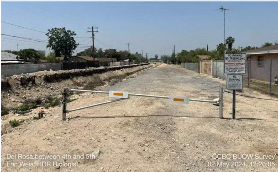
Photo 2. Looking W (downstream) along the City Creek Bypass Channel from the Del Rosa Dr crossing, between 4 th St and E 5 th St.
