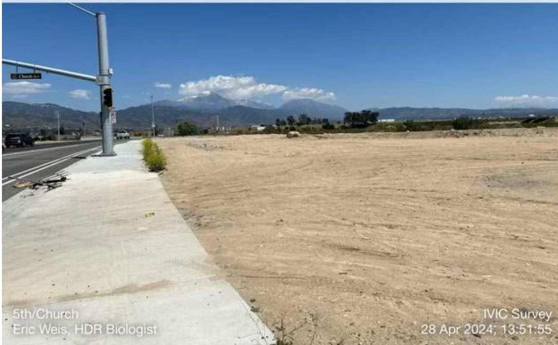
Photo 8. Looking E along 5 th St from the intersection of 5 th St and Church Ave.
