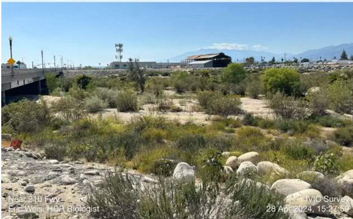
Photo 9. Looking W at City Creek from the NE corner of the 5 th St Bridge.
