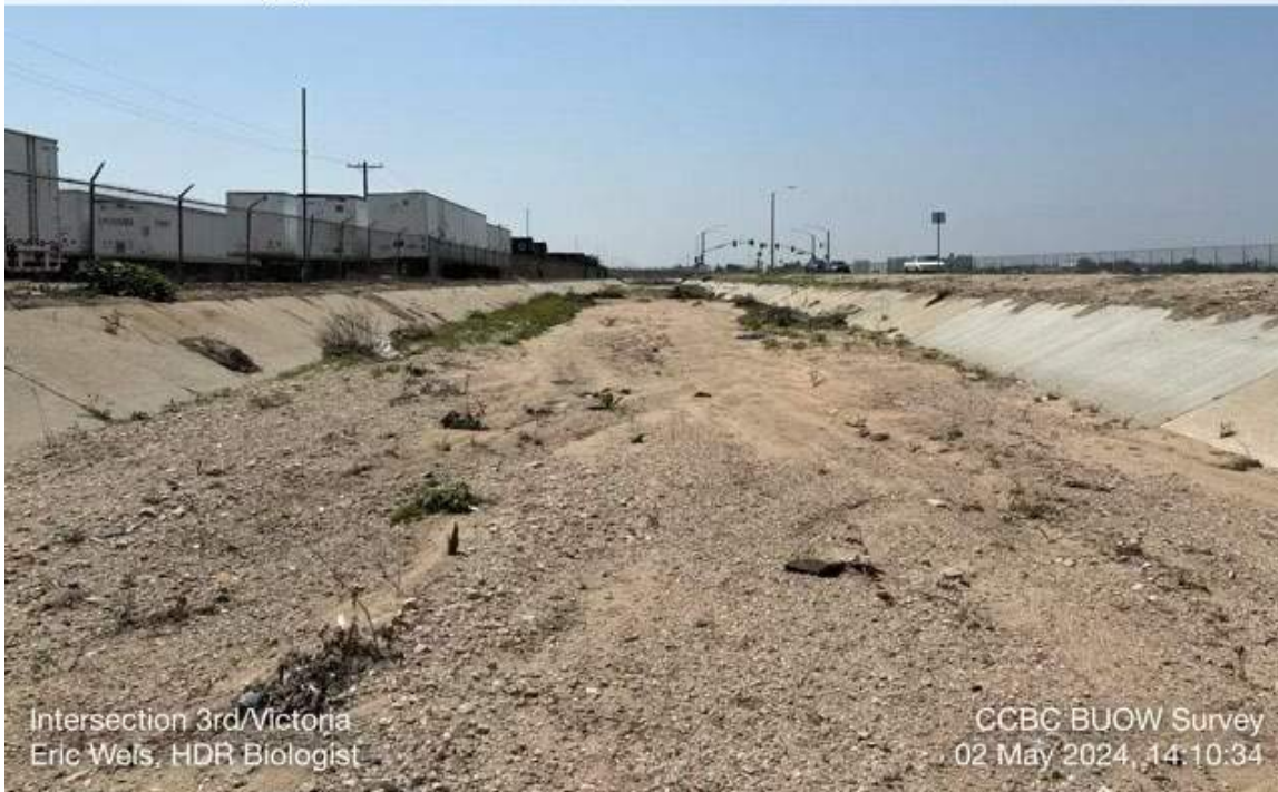
Photo 1. Looking W (downstream) along the City Creek Bypass Channel from the intersection of Victoria Ave and 3 rd St.
