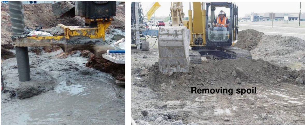
Image 39 – Deep soil mixing spoils: fresh (left side) and dried (right side).
