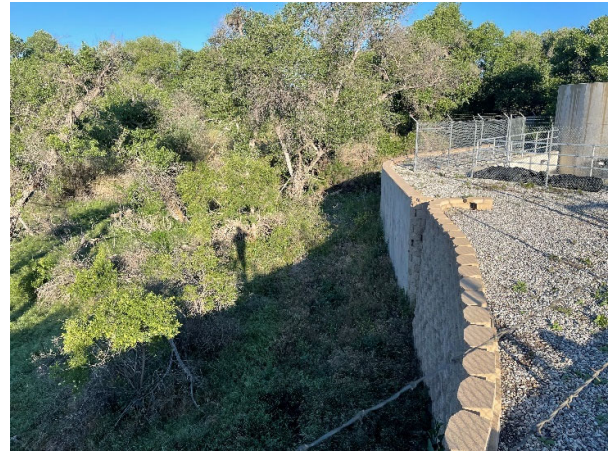
Image 3 – Transition from MSE wall to Cast-in-place wall, looking northwest
