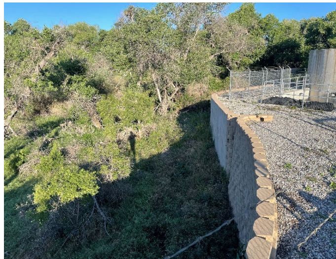
Image ES-2 –MSE wall and cast-in-place wall in the Middle Section, looking northwest
