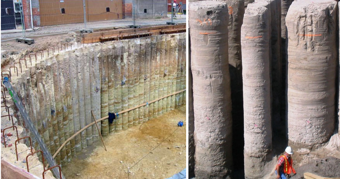
Image 15 – Examples of exposed Cement Deep Soil Mixing columns
