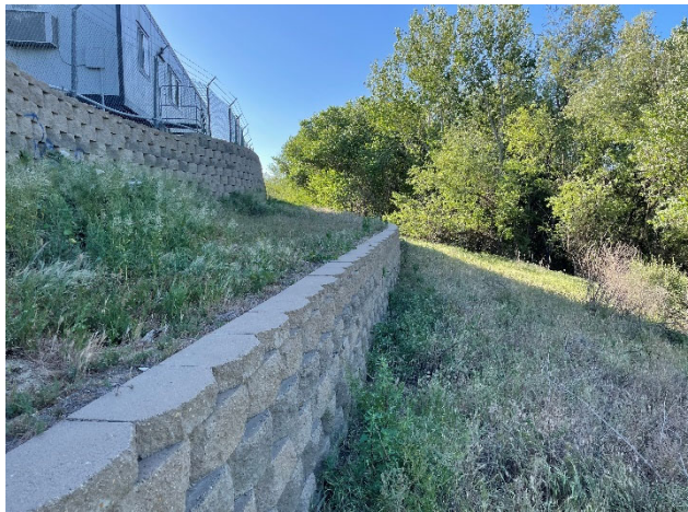
Image 4 – Existing two-tier MSE wall on southern end of the project area, left – aboveground visible portion; right – typical section;
