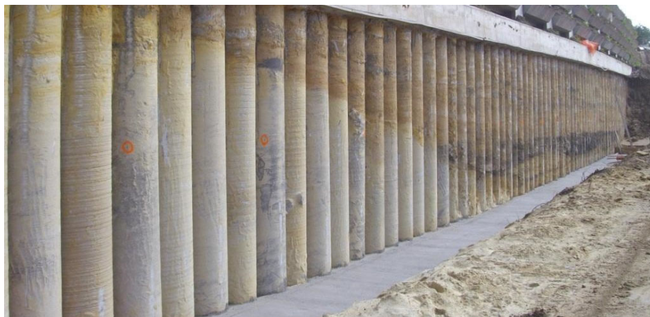
Image 19 – Examples of exposed secant pile wall
