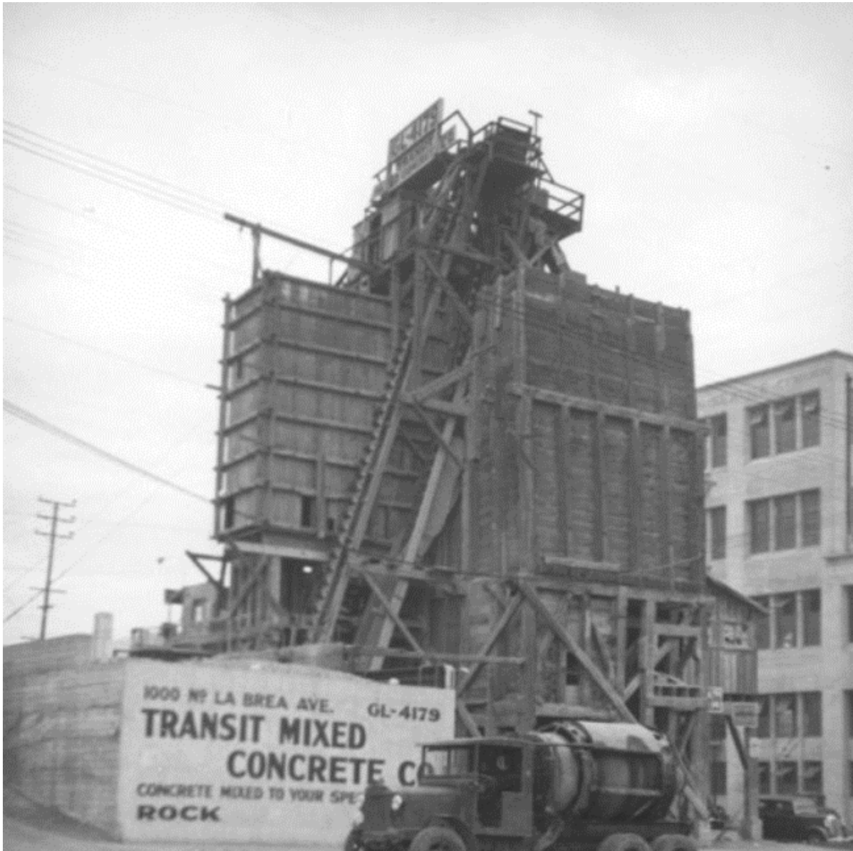
Figure 4.3-5 Mill and Truck Mixer at Transit Mixed Concrete Company, 1000 North La Brea Avenue, View to Southeast, 1937
