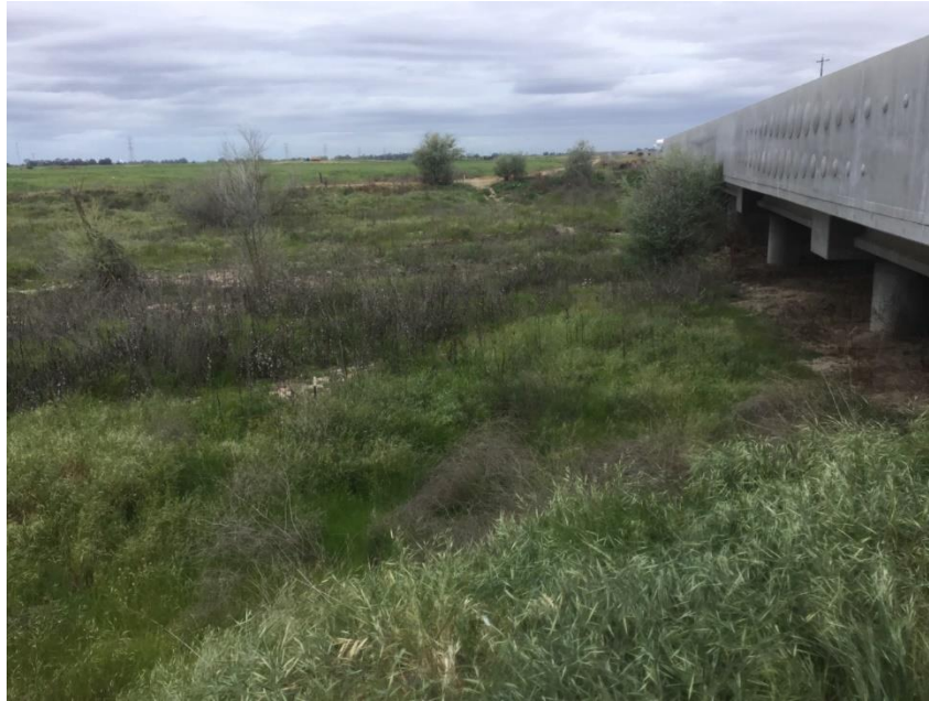
Photograph 3. Eastern side of Cottonwood Creek bridge, facing north (April 2024)
