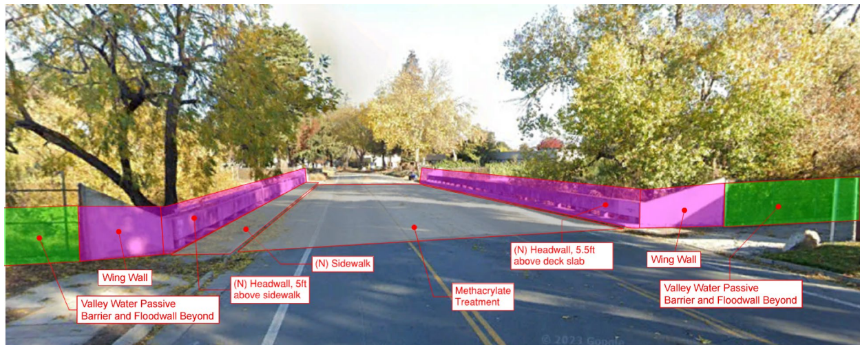
Figure 2.26. Charcot Avenue Headwalls and Wingwalls
