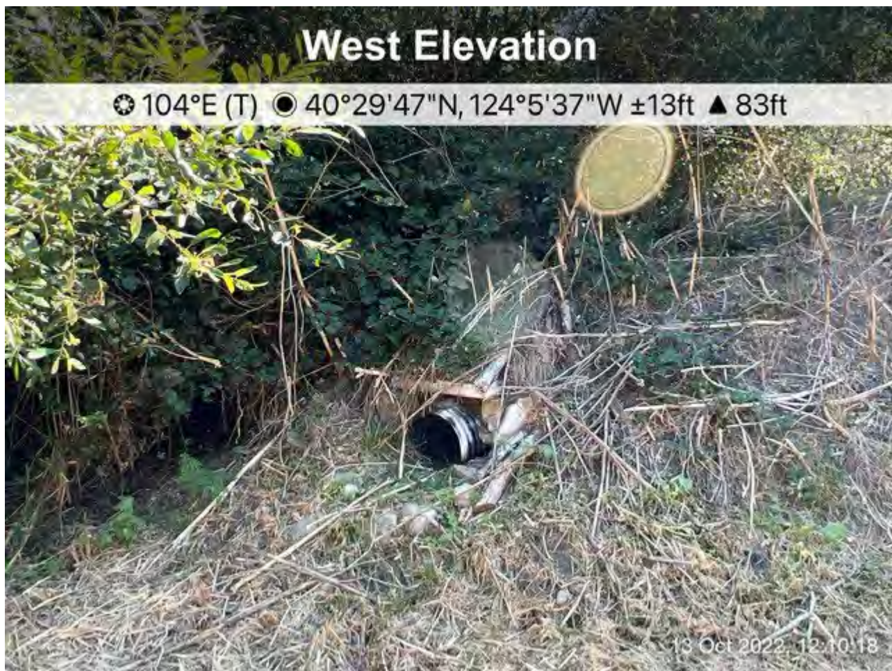
Photo 6. Overflow culvert in east bank of pond.
