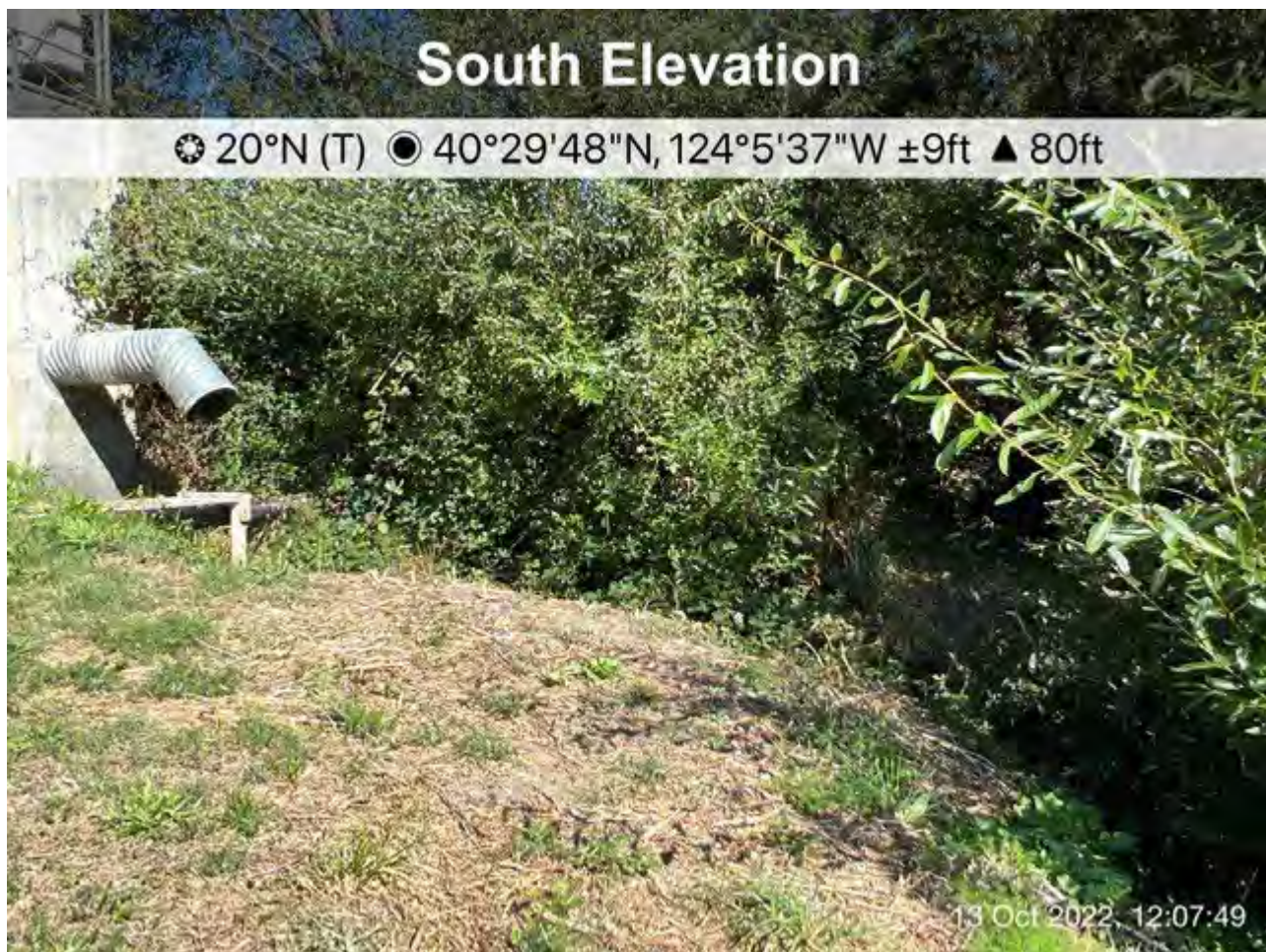
Photo 4. Outfall from the Rio Dell Treatment plant into Ditch 1, which flows into Wetland 1 on the right.
