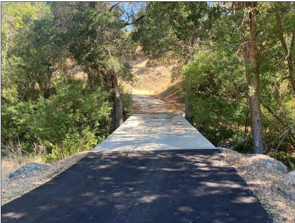
Photo 6. Bridge crossing at Tassajara Creek (aspect northeast; 9/1/22).
