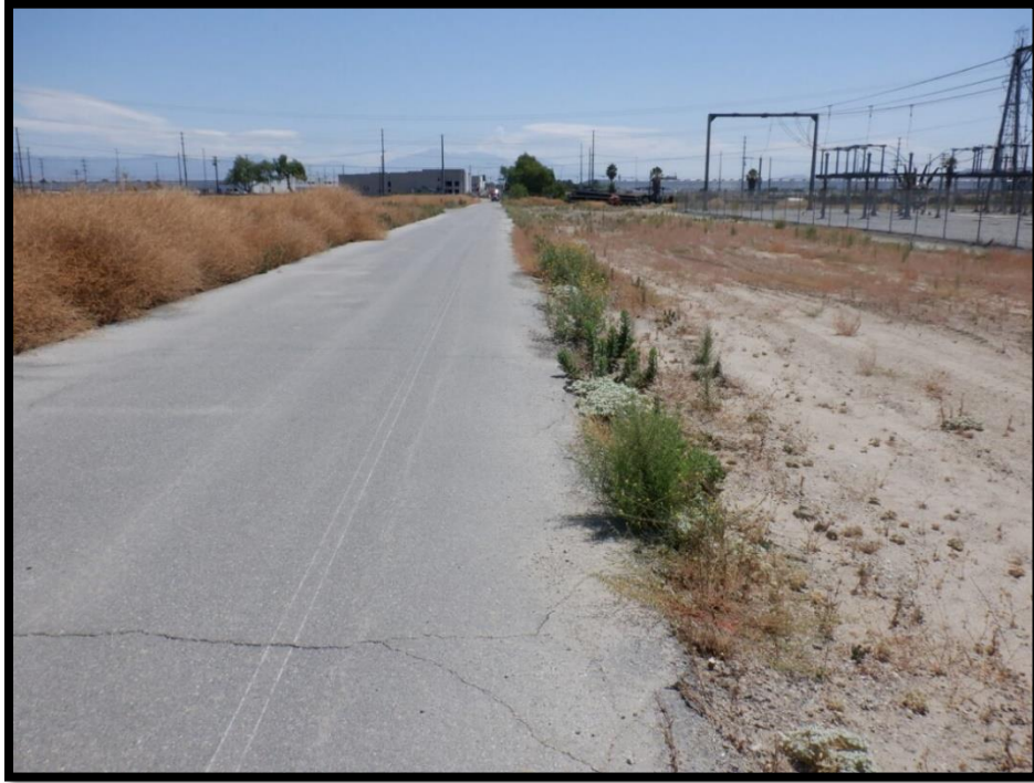
On Napa Road facing east in the southeastern side of the property. The entrance to the site is visible in the background. The median is on the left of the picture, the electrical substation is on the right.
