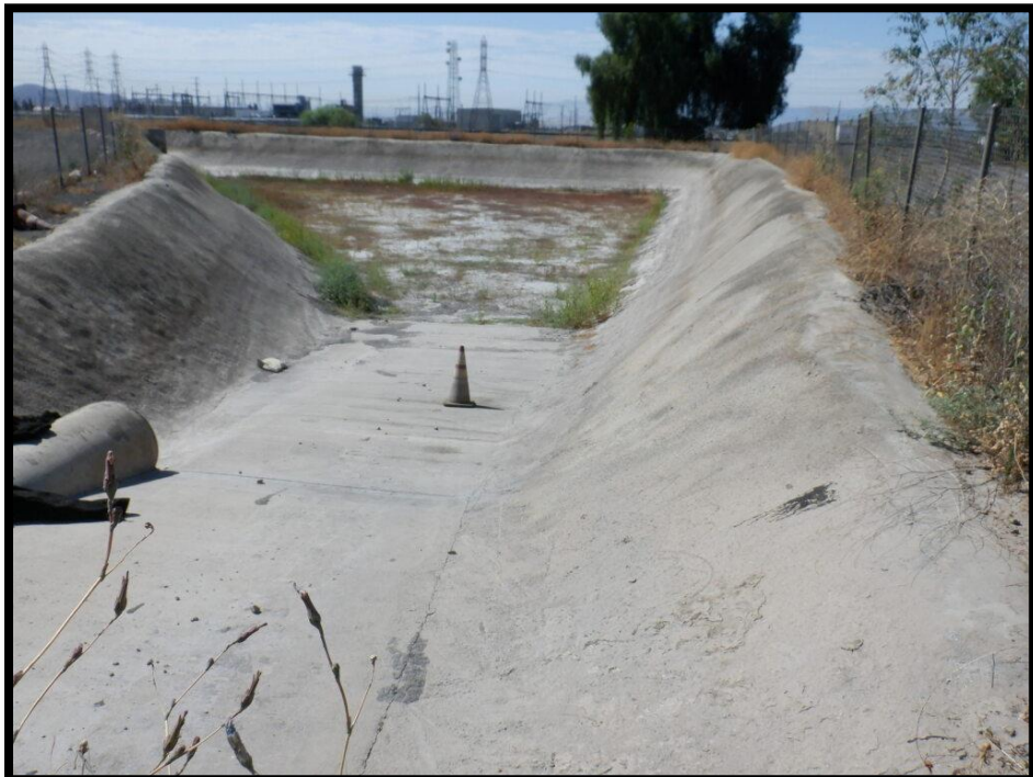
Looking into Basin 1 at the southwest end of the property. The shotcrete structure of the basin allows only for minimal vegetation growth.
