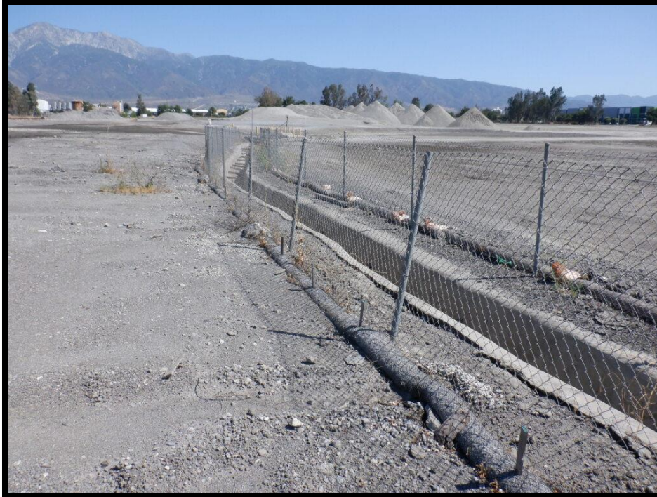
Looking north, a view of the channel associated with Basin 1 to help collect and direct surface water.
