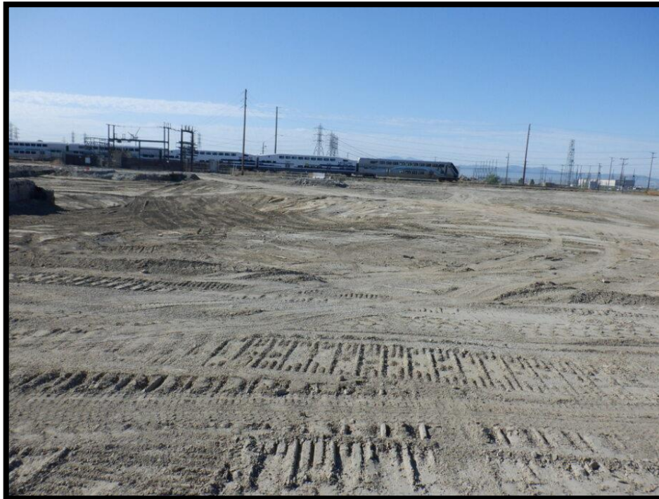
Looking south at the active Atchison Topeka and Santa Fe railroad, currently used by BNSF/Metrolink. Recent earthwork by heavy equipment is evident.
