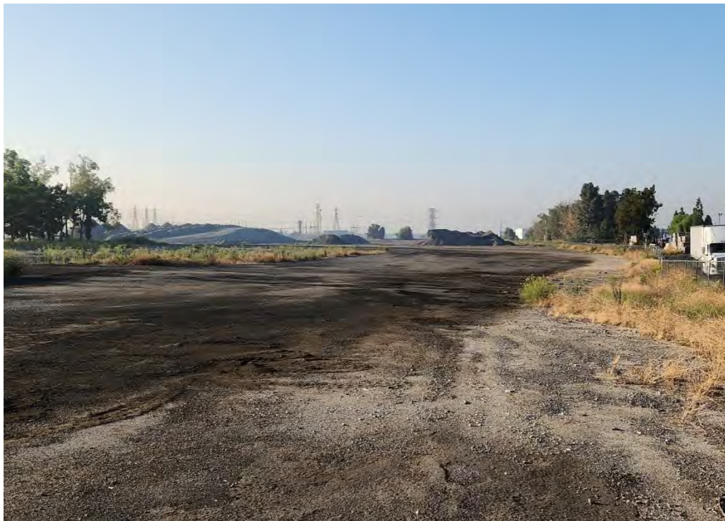
Figure 6. Oily sediments along western edge, sand and gravel piles in center of parcel, view to south.
