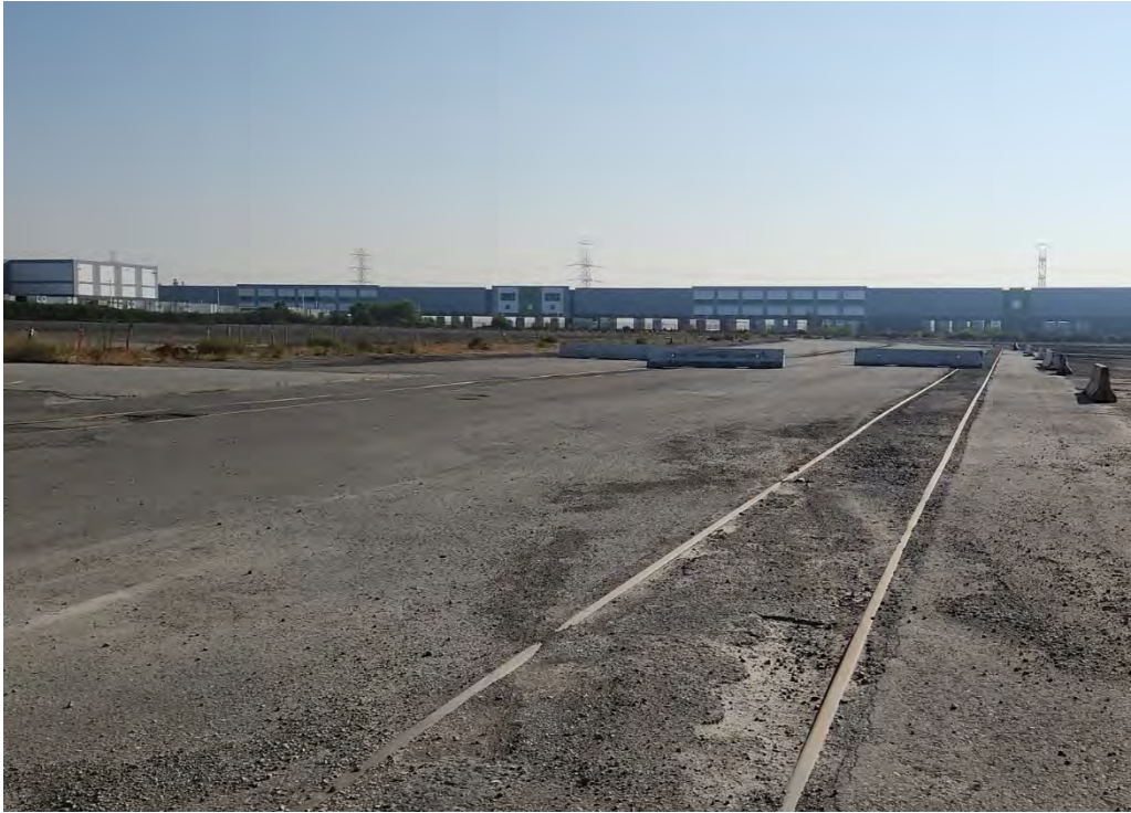
Figure 9. Northern portion of eastern 'arm' of parcel toward west building, view to east.
