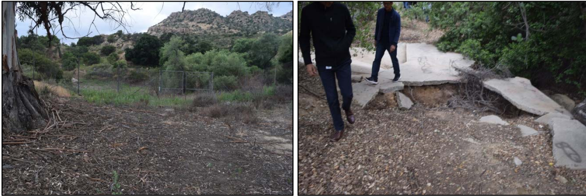
Figure 4 - Earthen Flood Control Basin and Broken Spillway
