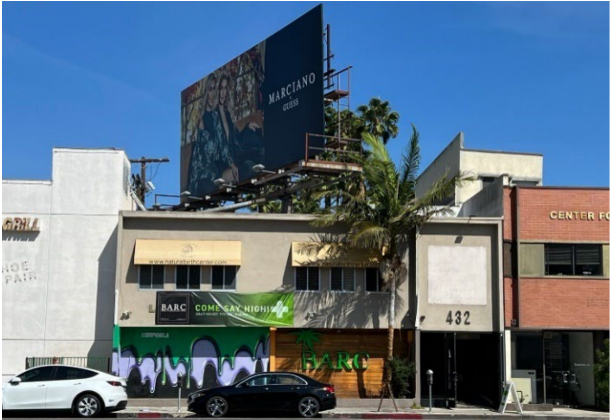
Figure 3: West elevation, view looking east. 2022. Source: GPA.
