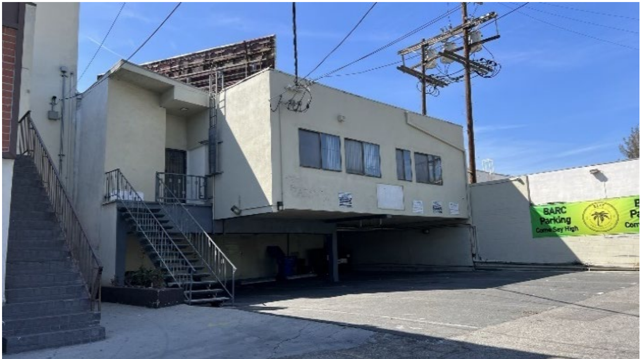
Figure 4: East elevation, view looking north. 2022. Source: GPA.
