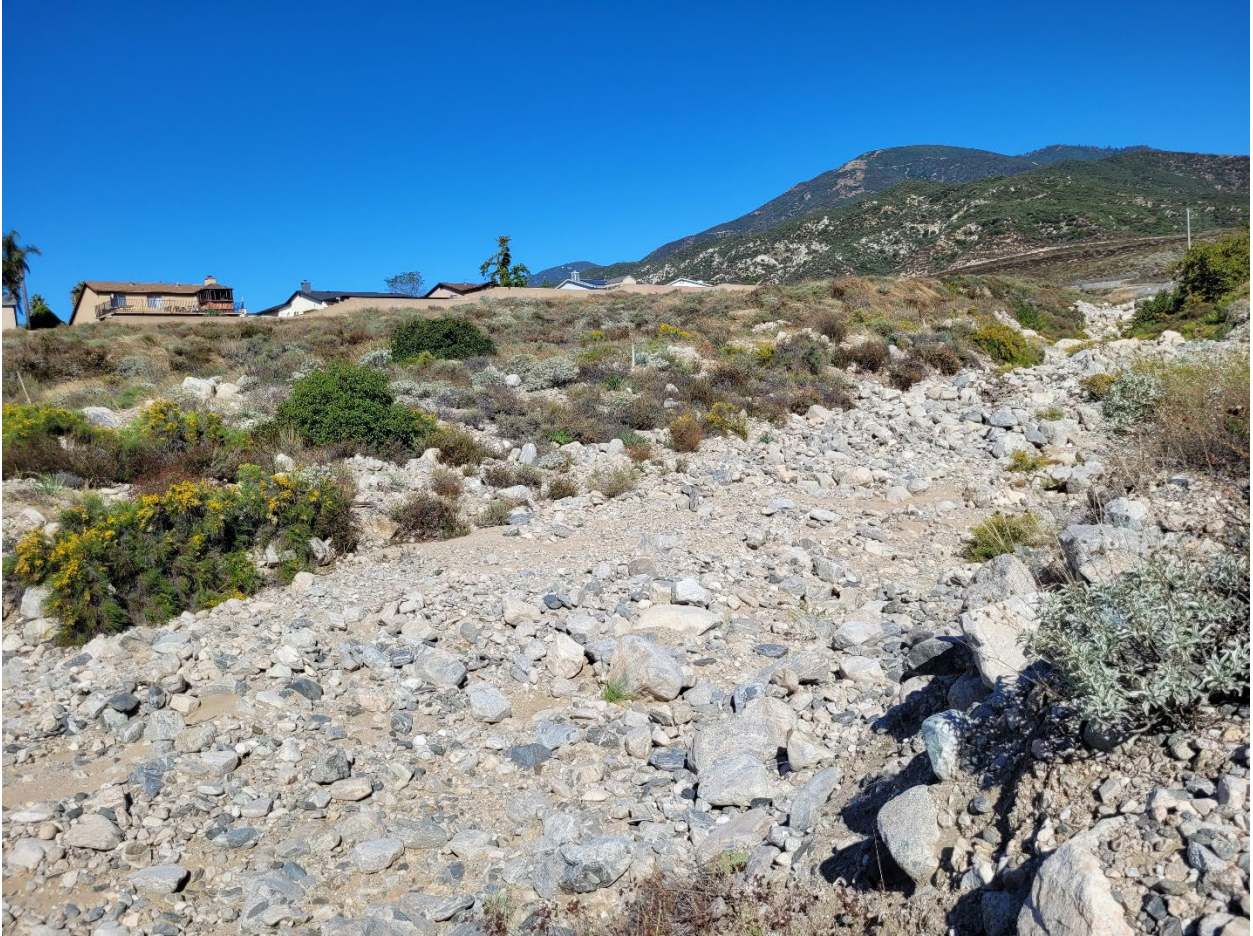
IMG 1: Rip-rap and vegetation along wasteway gates drainage path.
