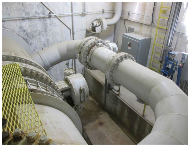
Figure B3 – Bypass Valve
