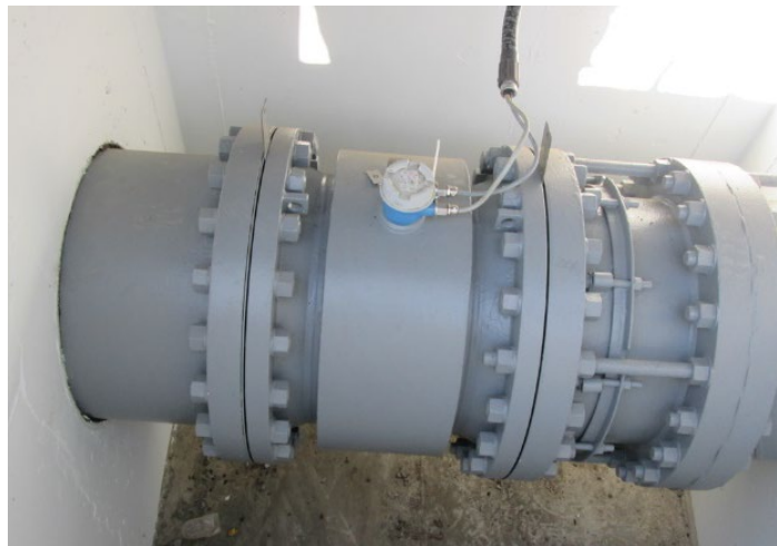
Figure C6 – Flow Meter
