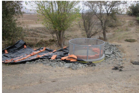
Figure F3 – Bank Stabilization and Erosion Control with visqueen BMP placed on top for dewatering.
