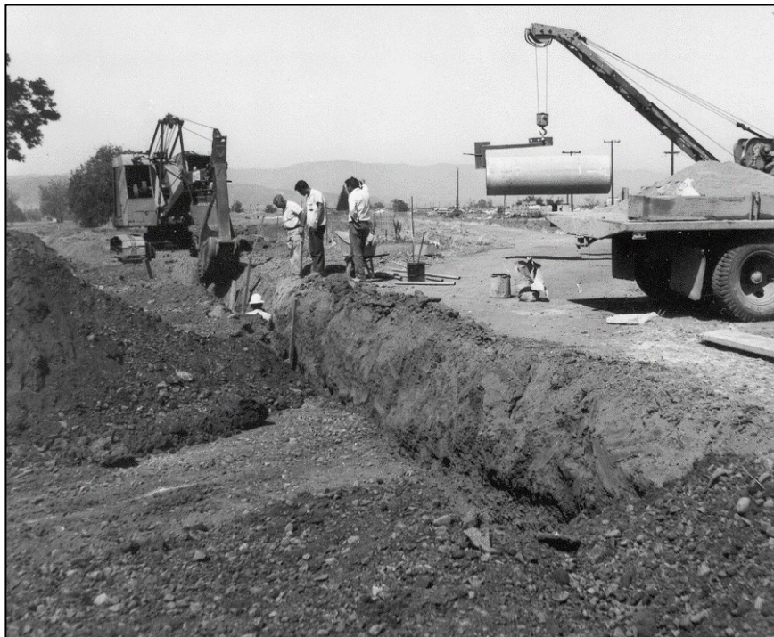
Plate 1. Alamitos Pipeline under construction in 1964 (courtesy of SCVWD Archives).
