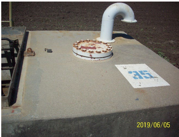
Figure E1 – Pump-out Riser
