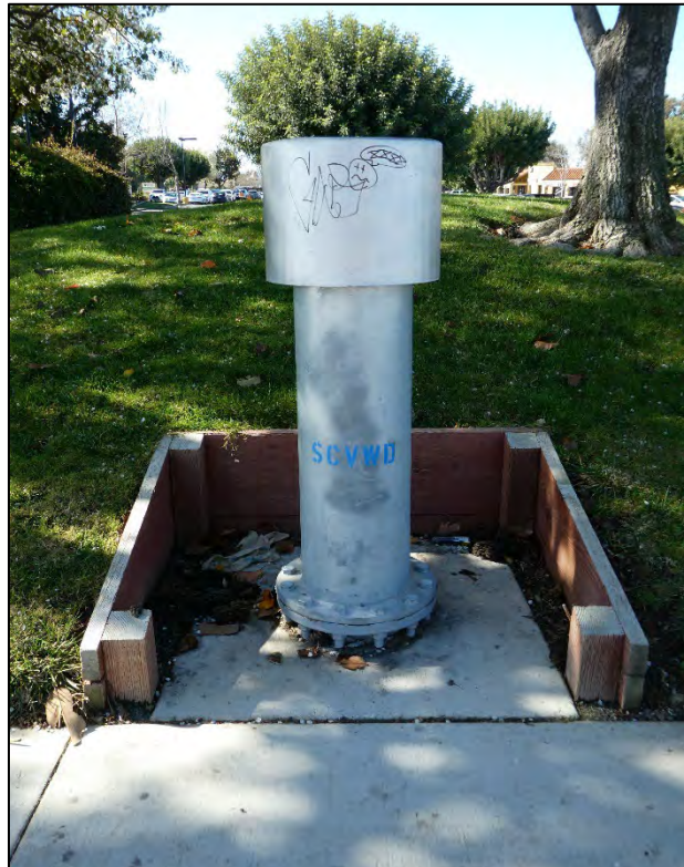
Photograph 9. Air vent on the East Pipeline, camera facing west, February 6, 2023.
