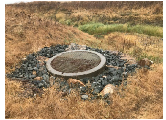
Figure E6 – Energy Dissipater
