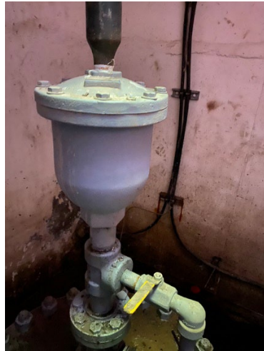
Figure B6 – Air Release Valve (ARV)
