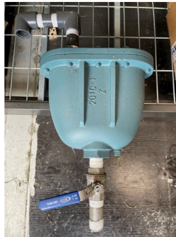
Figure B9 – Surge/Pressure Relief Valve
