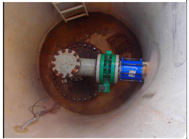
Figure B4 – Discharge/Blowoff Valve
