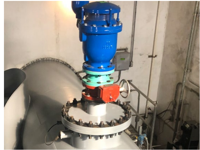
Figure B7 – Combination Air Release Valve (CARV)
