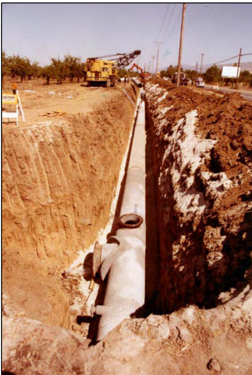
Plate 1. Two photographs of the East Pipeline under construction along North White Road in 1973 (courtesy of SCVWD Archives).
