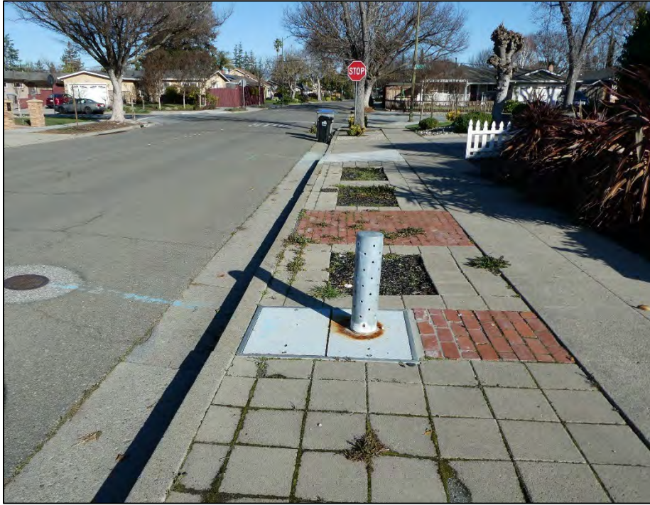
Photograph 2. Looking east along the right-of-way for the Campbell Distributary pipeline as it runs beneath a public street. An air vent is in the foreground. Photo taken February 6, 2023.
