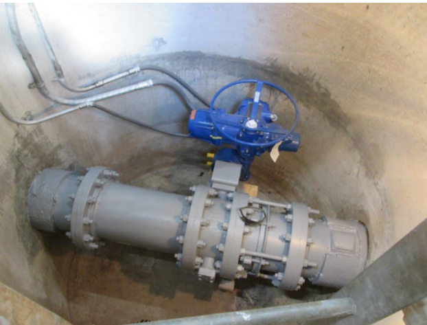
Figure B2 – Turnout and Modulation Valves
