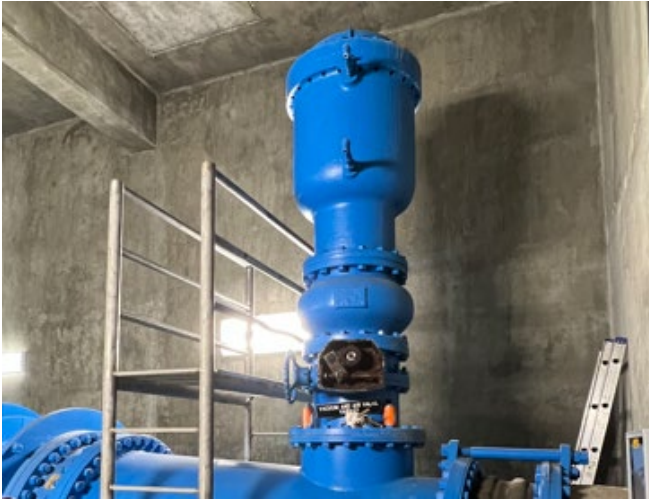
Figure B5 – Air and Vacuum Valve
