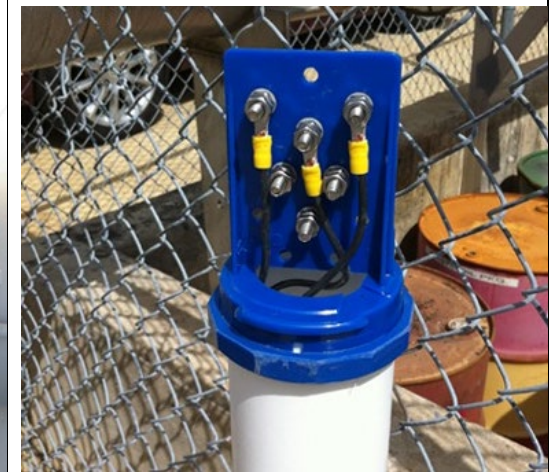
Figure D1 – Corrosion Control Test Station
