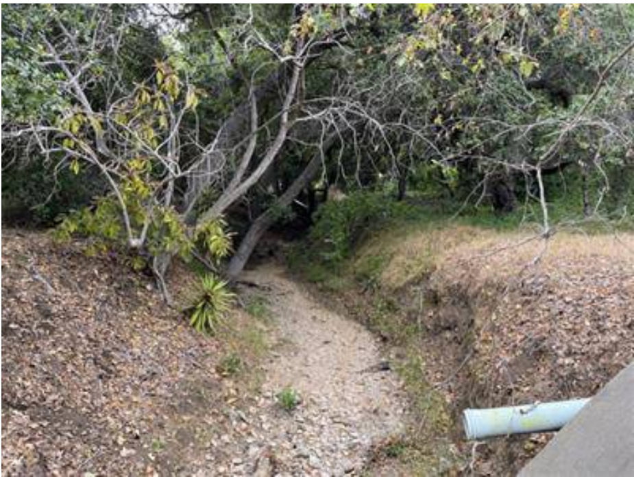
Photo Point 13 (facing north): Upstream view of drainage from bridge where channel passes through a culvert and then through a paved parking area.
