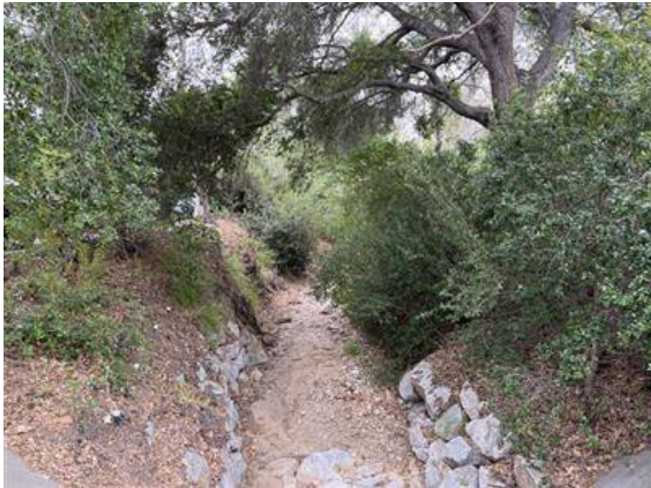
Photo Point 13 (facing south): Downstream view of partially reinforced channel after it passes through the culvert. Mature coast live oaks comprise the overstory tree layer.
