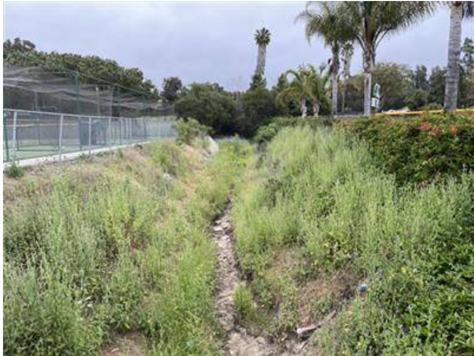
Photo Point 20 (facing north): Upstream view of reinforced channel running south to southwest from the catchment basin through the southern end of the project site; non-native tocalote dominant in the herbaceous layer.
