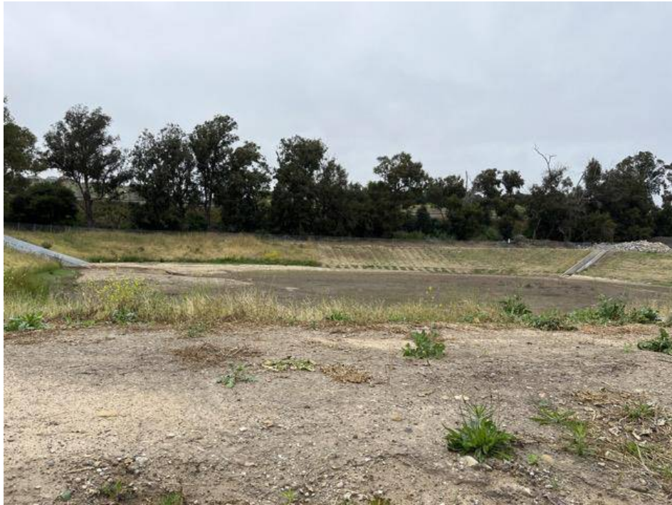
Photo Point 19 (facing north): View of debris and sediment management basin at southern end of property.
