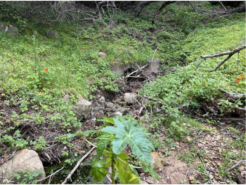
Photo Point 22 (facing south): Downstream view of drainage and culvert. Non-native castor bean ( Ricinus communis ) and nasturtium ( Tropaeolum majus ) visible.
