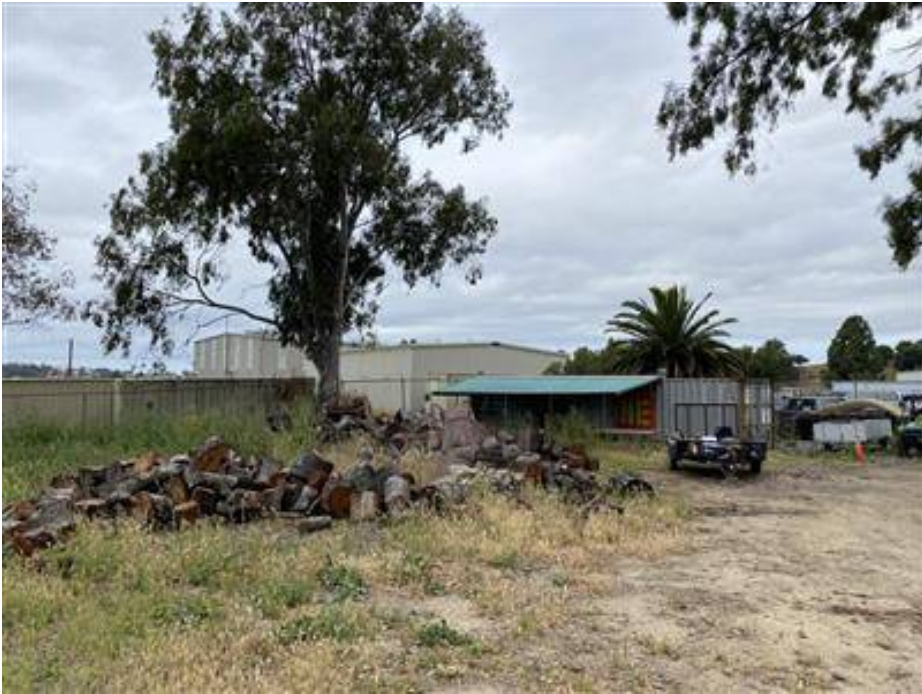
Photo Point 08 (facing east): Non-native landscape trees including Eucalyptus spp. and Canary Island date palm ( Phoenix canariensis ) growing adjacent to existing buildings planned for renovation or demolition.
