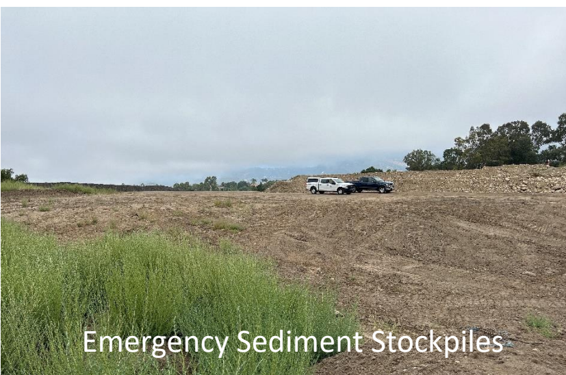
Emergency Sediment Ops
